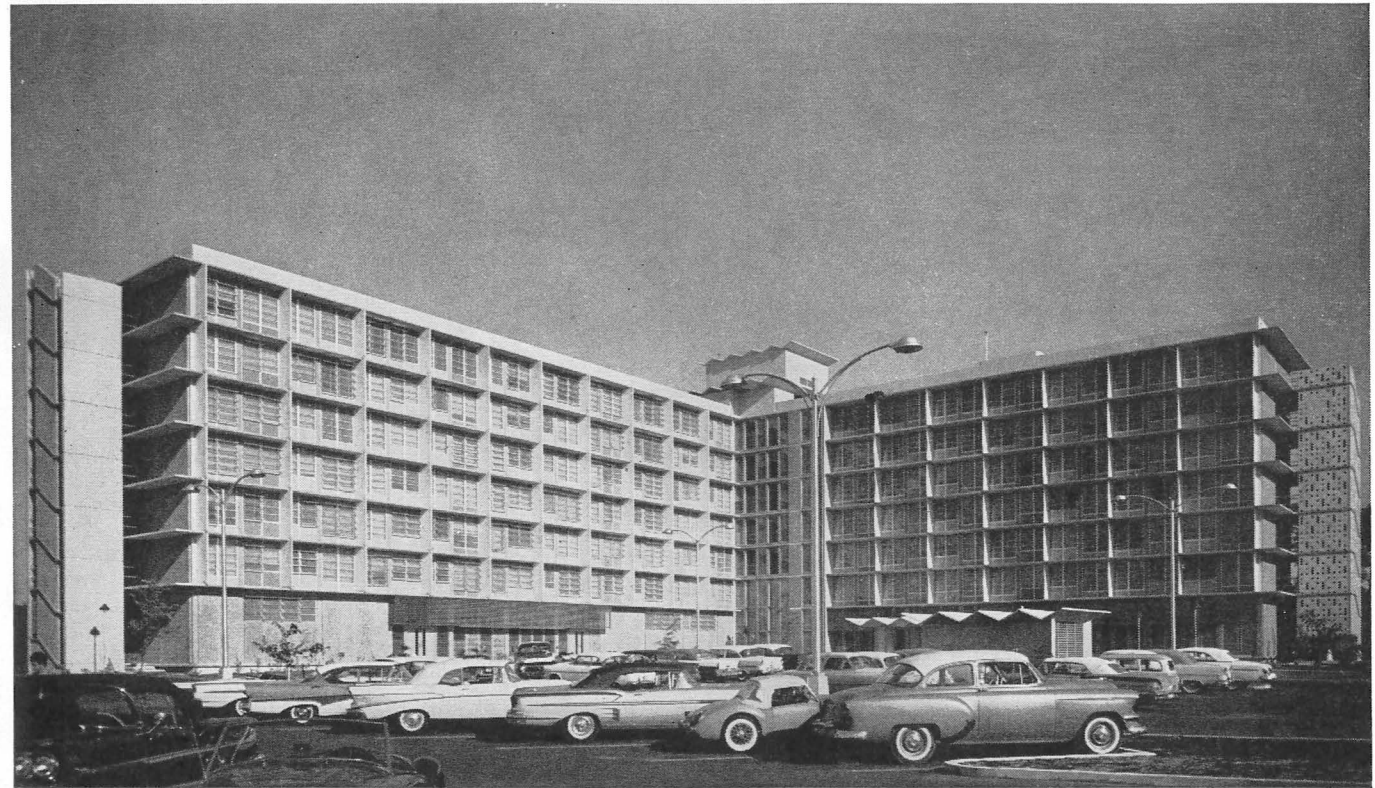
University of Miami Women's Dormitory • Robert M. Little, Architect J. E. Peabody, Norman J. Dignum, Engineers • M. R. Harrison Construction Co., Contractor
