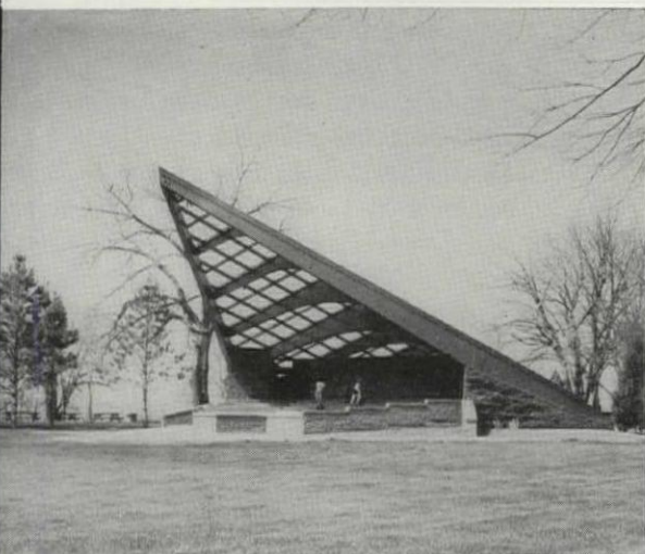
FIG. 2. ANOTHER OF THE ENDLESS VARIETY OF SHAPES AND FORMS POSSIBLE WITH GLUED LAMINATED TIMBER CONSTRUCTION IS ILLUSTRATED BY THE BANDSTAND IN TORRINGTON, WYO.
