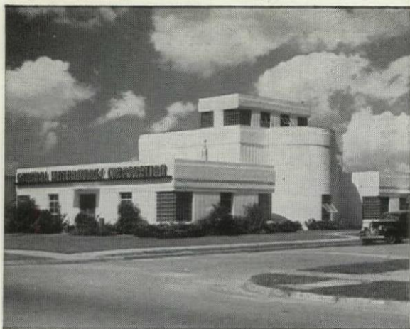
WATER WORKS, PINE BLUFF, ARK.
