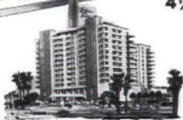
The Eden Roc , Miami Beach, Fla. Architect: Morris Lapidus, A.I.A. Contractor: Taylor Construction
