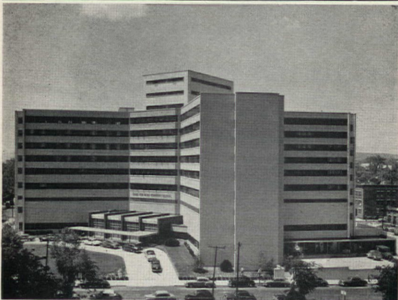
Memorial Unit — Grace-New Haven (Conn.) Community Hospital Architect — Office of Douglas Orr; Contractor — The Dwight Building Company
