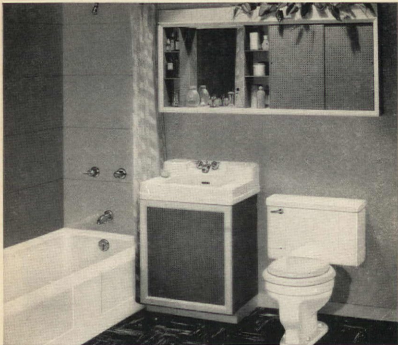
THIS PLEASING BATHROOM is only 5' x 7'. Note the use of a simple perforated wallboard enclosure to hide cleaning equipment under the lavatory. Crane fixtures, even in the low-priced lines, feature clean, modern styling.
