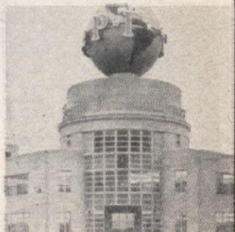
POST-INTELLIGENCER, Seattle Wash. Arm-Glaze used throughout. Architectural Consultant, Rusty Dittman; Gen. Contractor, Howard S. Wright & Co.; Engineers, Lockwood Greene Inc.; Glazing Contractor, W. P. Fuller & Co.
