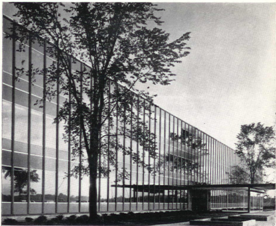
ENGINEERING STAFF BUILDING, GENERAL MOTORS TECHNICAL CENTER, NORTH OF DETROIT, MICH.
