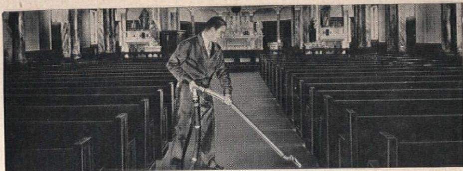
The vacuum producer and dirt container are located in the basement. Piping connects to convenient inlets all over the building.
