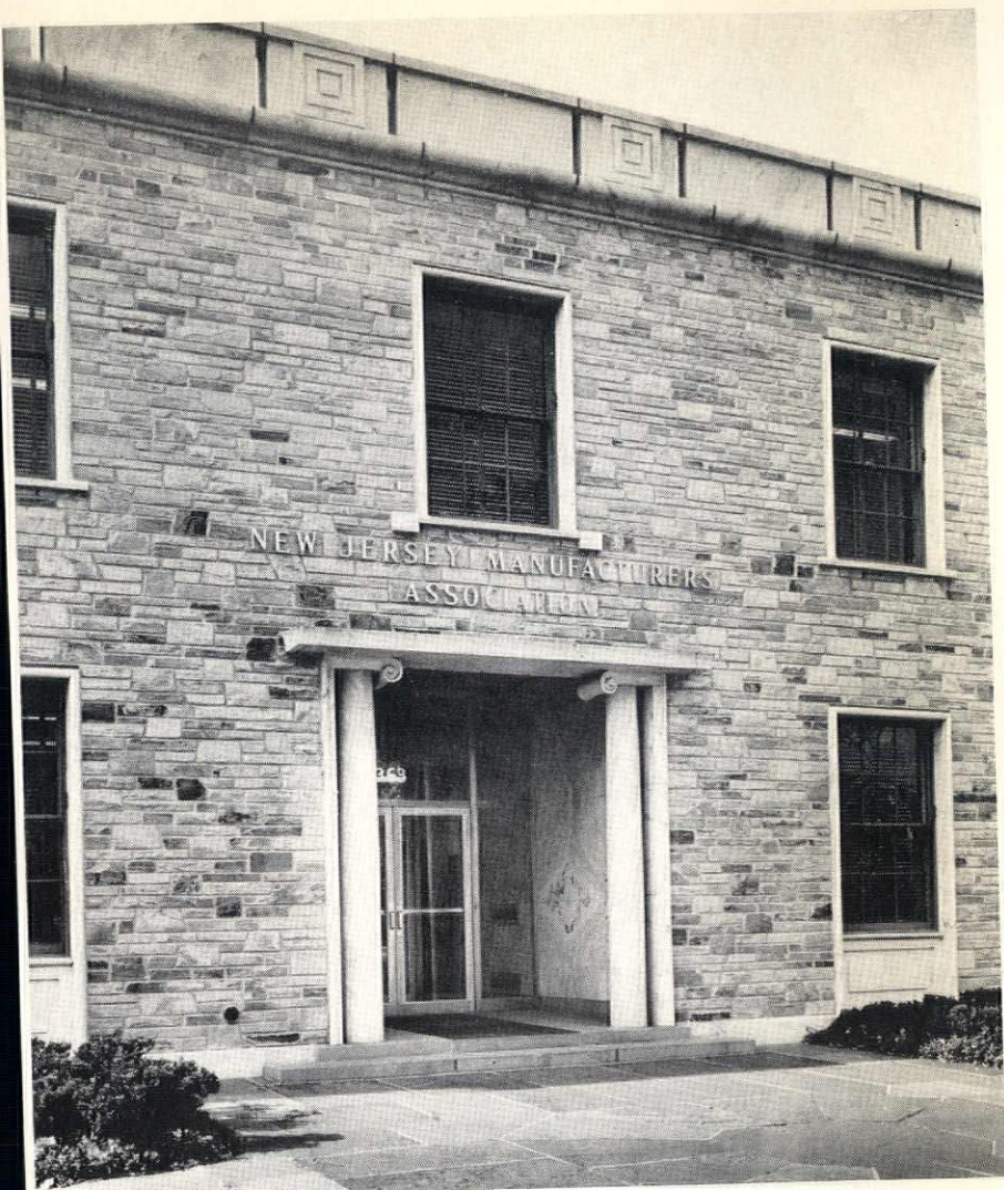
ENTRANCE DETAIL. NEW JERSEY MANUFACTURERS' ASSOCIATION BUILDING TRENTON, NEW JERSEY
