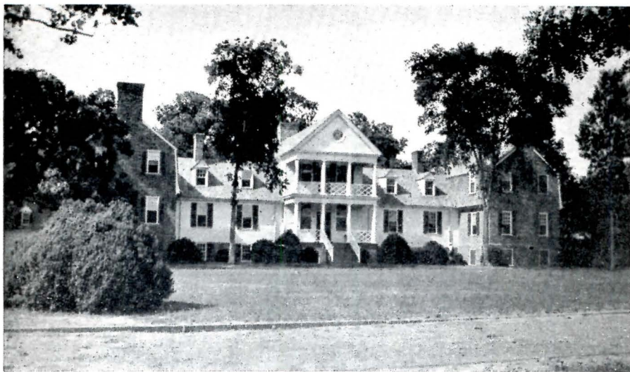
REMODELED COUNTRY HOUSE OF COL. HENRY ANDERSON, DINWIDDIE COUNTY, VA.
