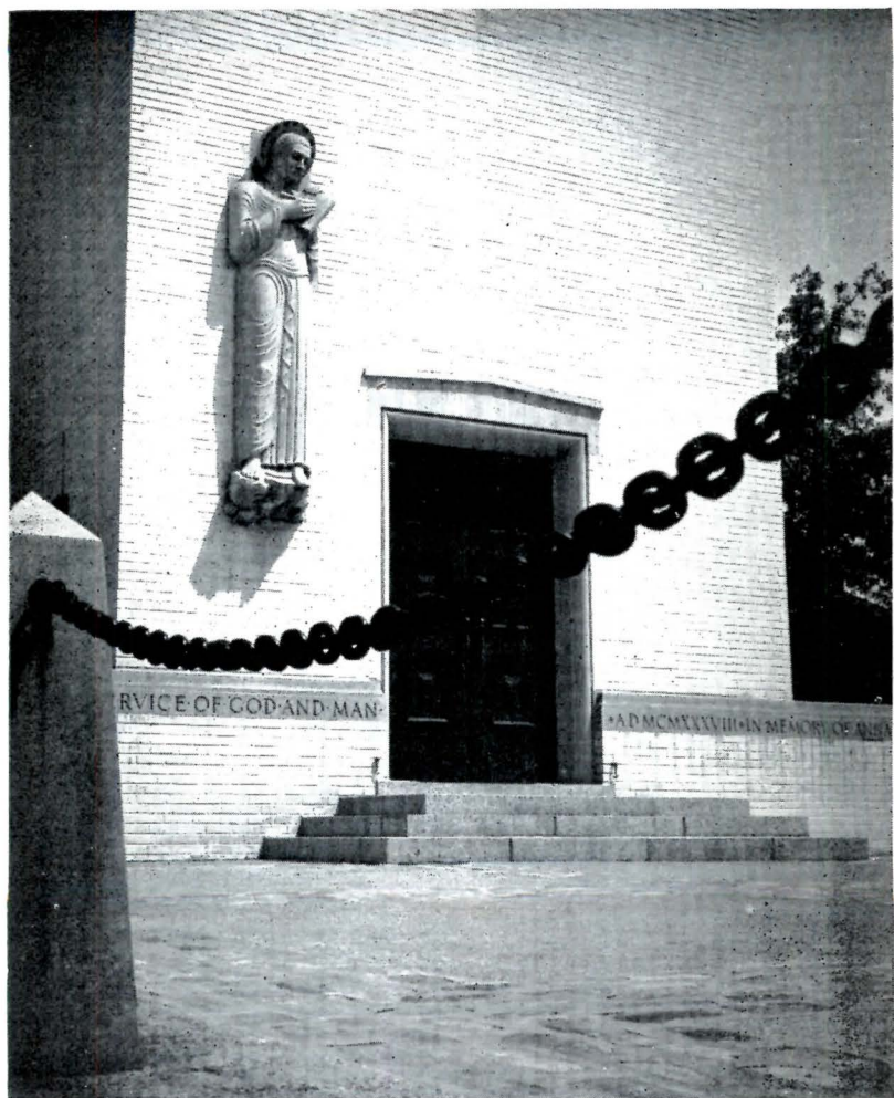
DETAIL OF WEST FRONT THE PROTESTANT EPISCOPAL CHURCH OF ST. MARK'S, ST. LOUIS, MO. NAGEL & DUNN, ARCHITECTS
