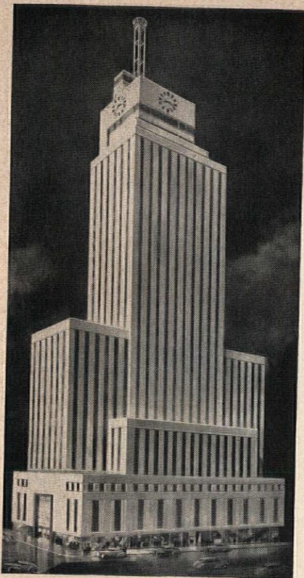
"City in the Sky"--the Mercantile Bank Building, Dallas, Texas. Youngstown Pipe used for plumbing, heating and air-conditioning. Architect, Walter W. Ahlschlager, general contractor, Henger Construction Co., plumbing sub-contractor, C. Wallace Plumbing Co.--all of Dallas.
