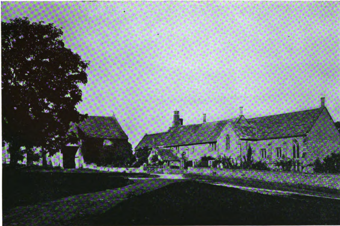
PRESTON BERMONDSEY, YEOVIL, SOMERSETSHIRE
