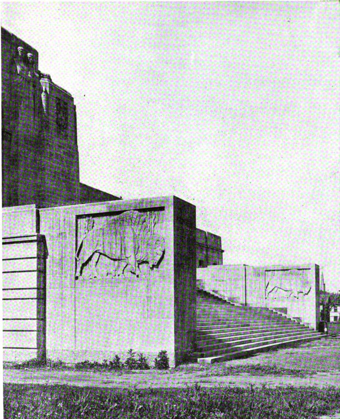
BALUSTRADE AND STEPS—MAIN ENTRANCE
