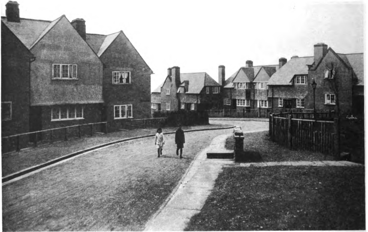
GOVERNMENT HOUSING SCHEME, WELL HALL, WOOLWICH. 1915. WHINYATES ROAD from ROSS WAY Looking South.
