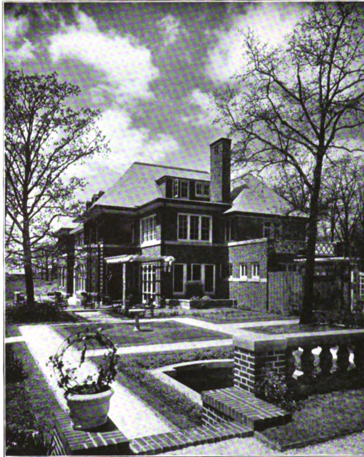
Residence Arthur H. Fuerbacher, Esq., Saint Louis Co., Missouri M. P. McArdle, Architect Hy-tex Velour Matts, Flemish Bond with 1/2-inch gray, tooled mortar joint
