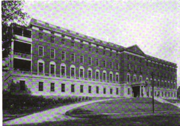
Mt. Sinai Hospital, Cleveland, Ohio G. B. Post & Son Co., Architects
