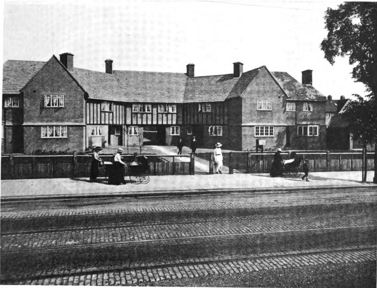
GOVERNMENT HOUSING SCHEME, WELL HALL, WOOLWICH. 1915. Entrance Group in WELL HALL ROAD, East Side.
