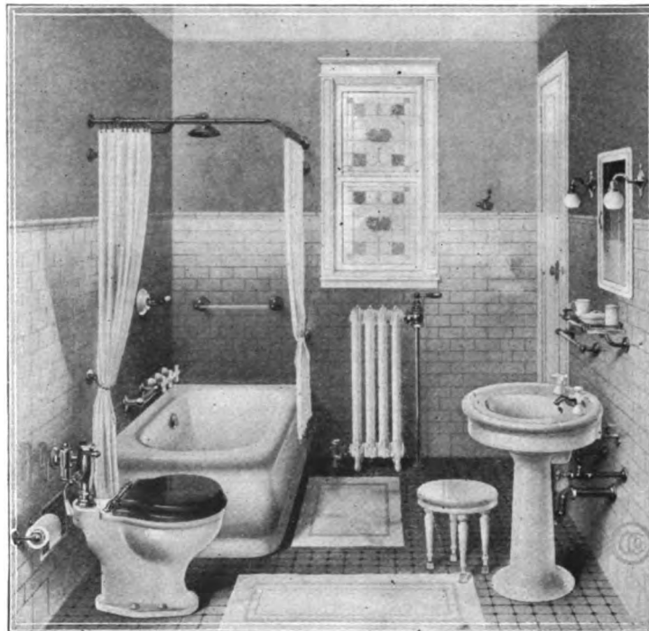
Typical CRANE Bathroom
