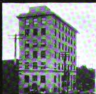
American Bank Building Suffolk, Va.
