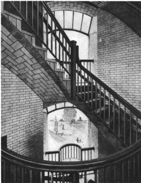
NON-COMMUNICATING ECONOMIC OPEN STAIRS, WEATHER PROTECTED. INTERCOMMUNICATION, INFECTION AND CONTAGION REDUCED TO A MINIMUM
