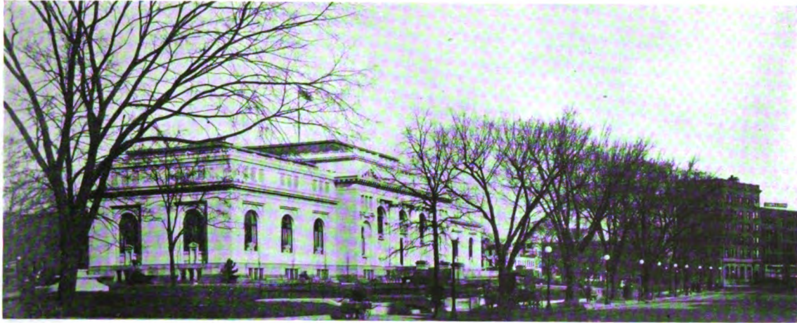
FIGURE 13. SOUTH SIDE OF WASHINGTON PUBLIC LIBRARY. Mounting Height of Lights, 12 Feet
