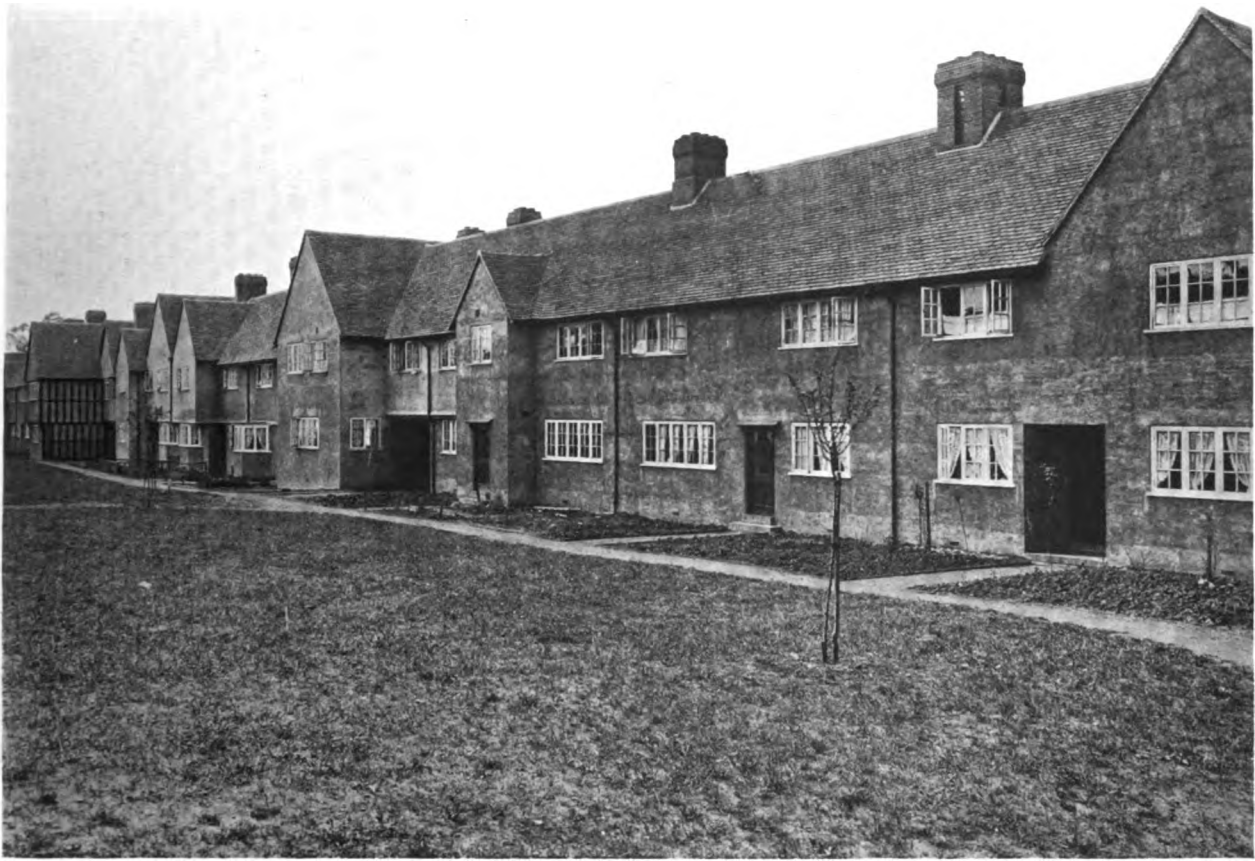
GOVERNMENT HOUSING SCHEME, WELL HALL, WOOLWICH. 1915. A Group in WELL HALL ROAD Looking South.
