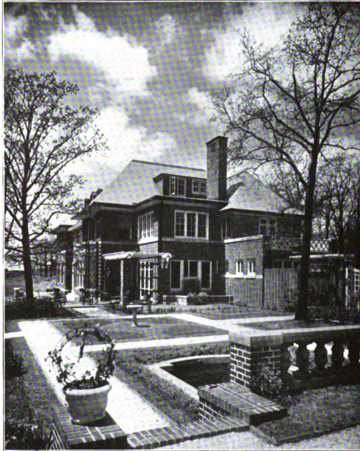
Residence Arthur H. Fuerbacher, Esq., Saint Louis Co., Missouri M. P. McArdle, Architect Hy-tex Velour Matts, Flemish Bond with 1/2-inch gray, tooled mortar joint
