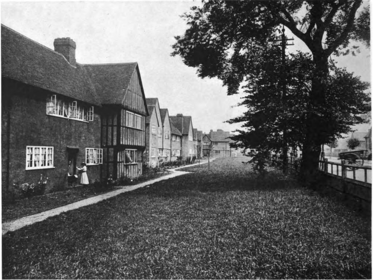
GOVERNMENT HOUSING SCHEME, WELL HALL, WOOLWICH. 1915. View in WELL HALL ROAD Looking North.
