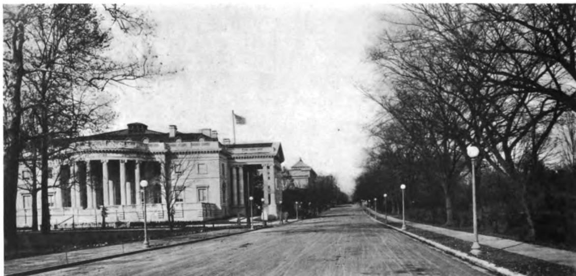
FIGURE 12. SEVENTEENTH STREET. MEMORIAL HALL OF THE DAUGHTERS OF THE AMERICAN REVOLUTION IN FOREGROUND. Lamps Staggered, 60 Feet Spacing, Mounting Height 12 Feet, Roadway 50 Feet
