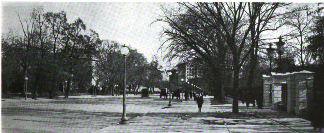
FIGURES 8-9. PENNSYLVANIA AVENUE AT THE WHITE HOUSE. LAMPS IN PAIRS (PARALLEL ARRANGEMENT). Mounting Height of Lights, 12 Feet, Roadway 80 Feet
