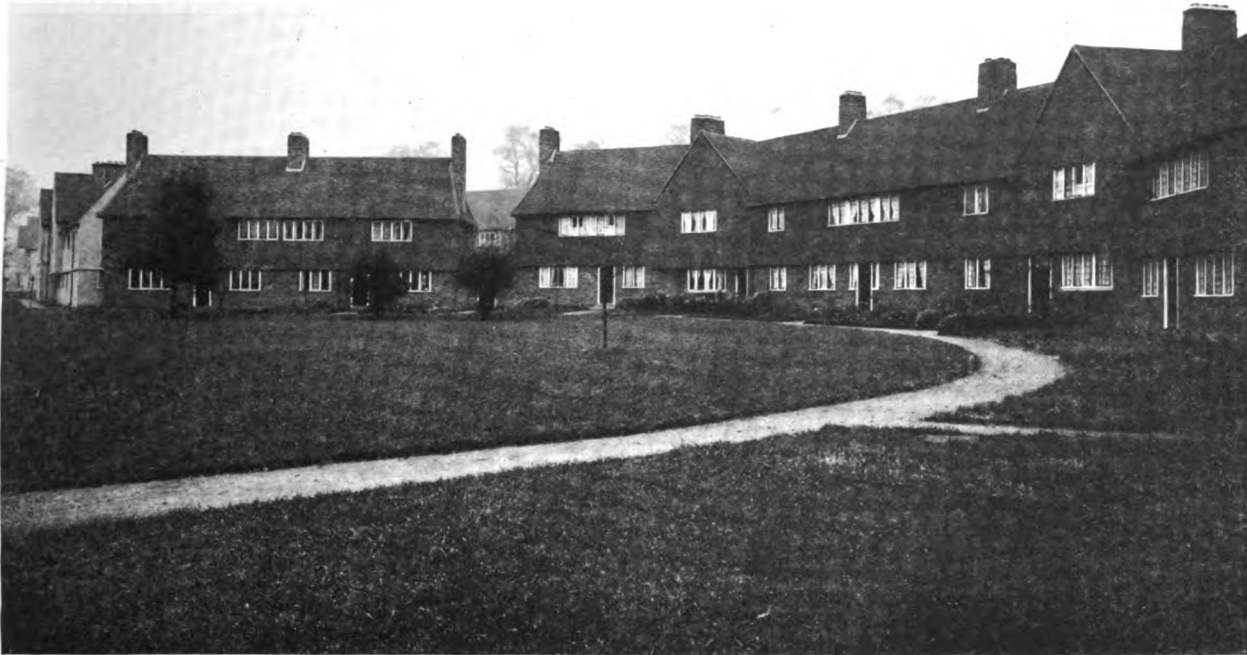
GOVERNMENT HOUSING SCHEME, WELL HALL, WOOLWICH. 1915. Crescent near Station in WELL HALL ROAD.
