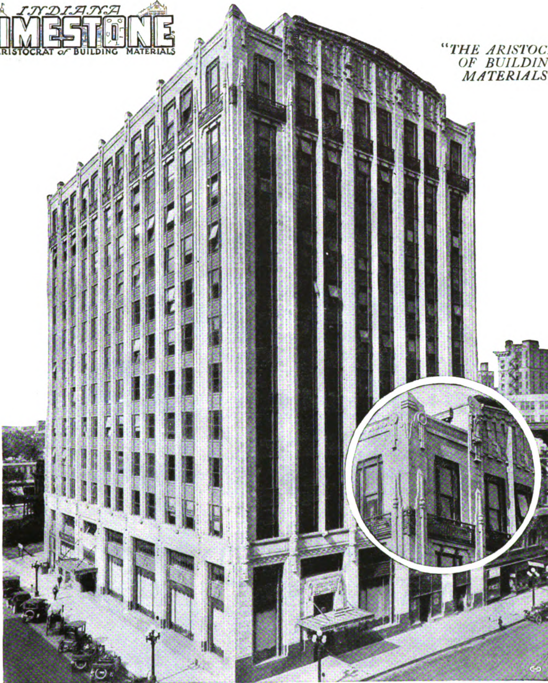
Metropolitan National Bank Building, Minneapolis: Masonry of all fronts is Indiana Limestone. Hewitt & Brown, Architects.
