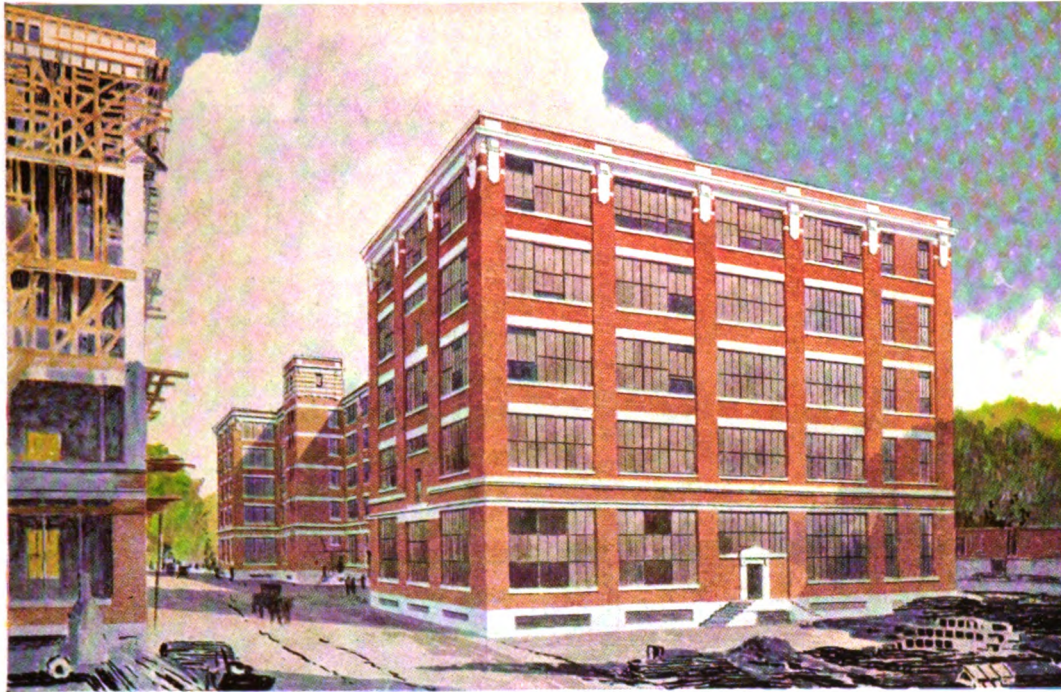
General Electric Company, Fort Wayne, Ind. Harris & Richards, Architects Structural concrete building faced with brick
