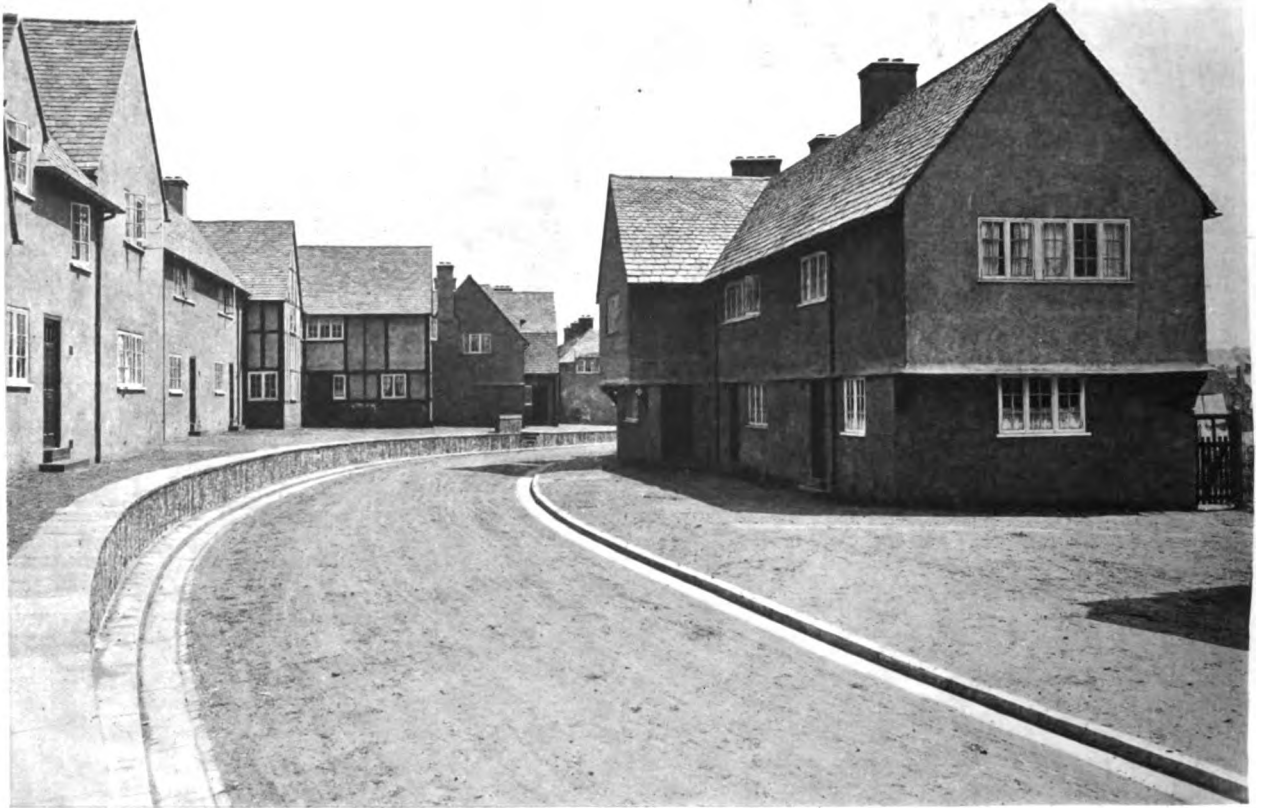
GOVERNMENT HOUSING SCHEME, WELL HALL, WOOLWICH. 1915. View in ROSS WAY Looking East.
