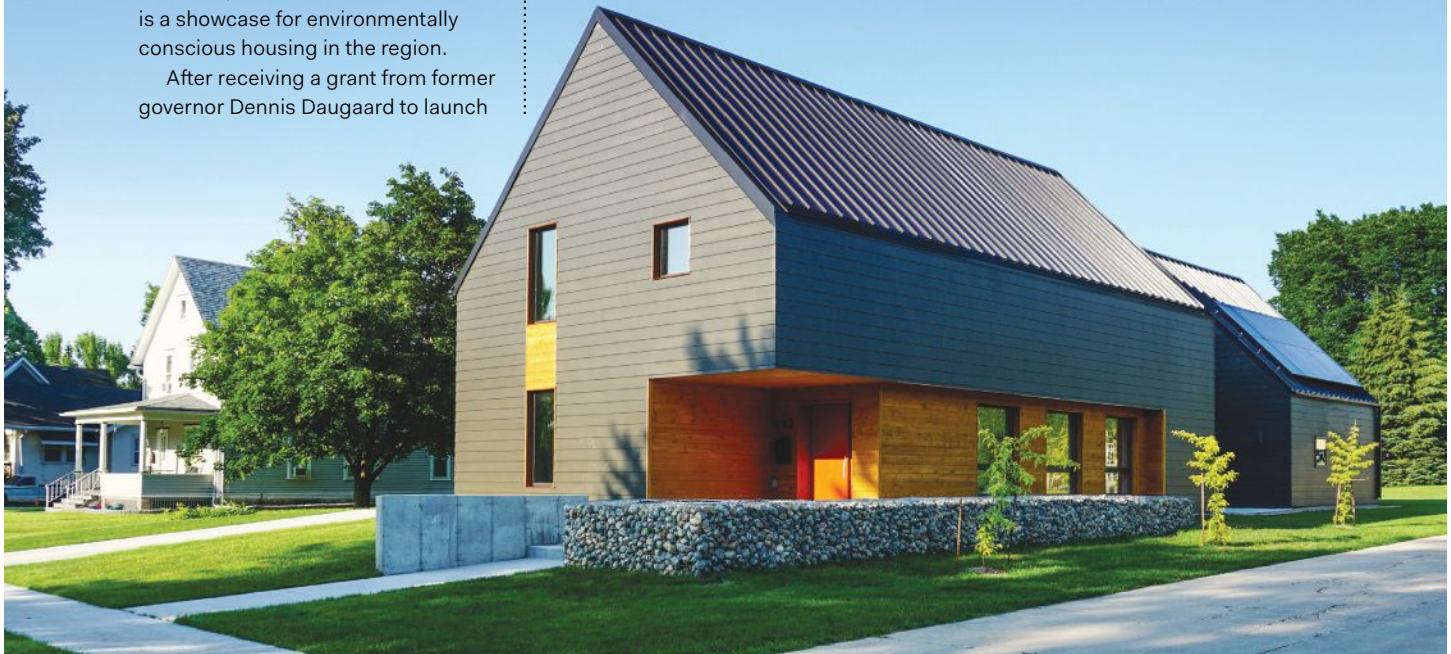
Cement-fiber lap siding conceals Zip System sheathing from Huber.
