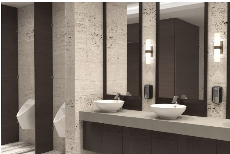
Anything that eliminates or reduces the number of surfaces the user touches cuts down the potential for cross-contamination. Sensor-operated restroom fixtures that prevent the need to touch surfaces are an important component of hygienic restroom design.
