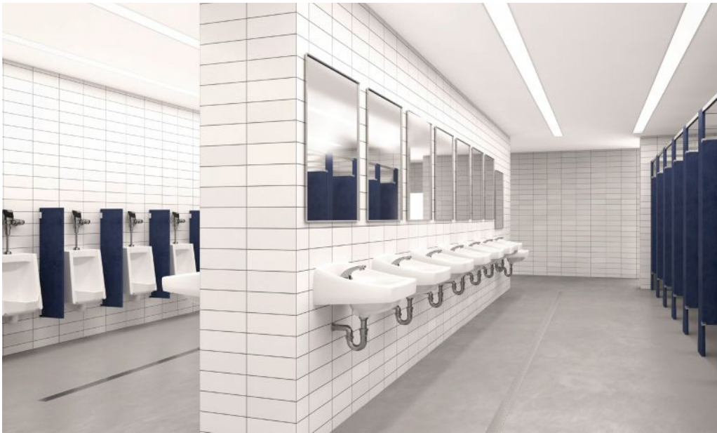
Using wall-hung vitreous china lavatories is a cost-saving option that allows some schools to utilize higher-tech sensor faucets and flushometers to still achieve improved hygiene and convenience. Photo courtesy of Sloan Valve Company
