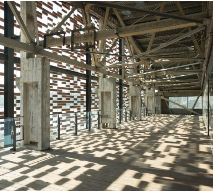
Suspended Brick Façade Detail
