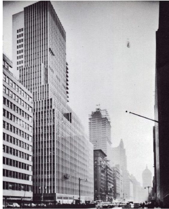
425 Park, currently being redeveloped by Foster + Partners
