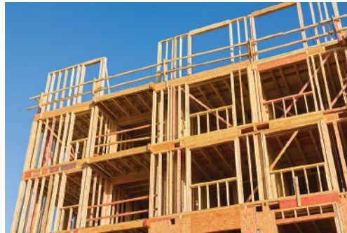
Light frame wood construction has long been the go-to framing choice for low-rise and, increasingly, mid-rise residential and commercial buildings.
