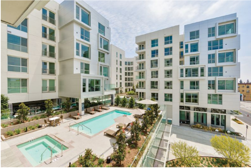
Tenants are seeking green space such as an atrium, courtyard, rooftop patio and/or pools; podium and wrap construction make this possible. WREN | Architect: Togawa Smith Martin, Inc. | Photo: Kevin C. Korczyk
