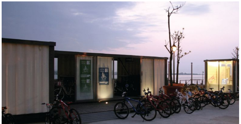
Taipei-based B+P Architects’ recent design for a shipping-container art annex in New Taipei City is a nod to the city’s multiphase port expansion that began in 1993.
