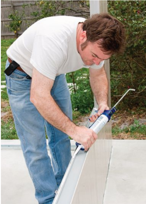
ASTM C 920 defines a joint sealant using several descriptor categories. For example, this sealant would be a Type S: Single component, Grade NS: Non-sag product.
