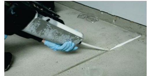
Two component polyurea based joint sealants are applied using specialized plural component equipment and cure quickly to reduce downtime.
