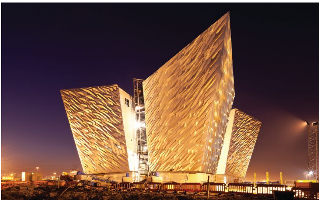
Titanic Belfast, Belfast, Northern Ireland. Photo courtesy of Kingspan Insulation LLC.
