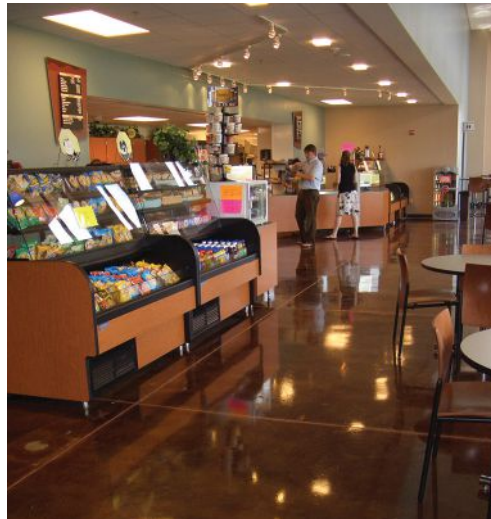
This floor coating was completed in the summer of 2007, demonstrating the long term durability of this technology.
