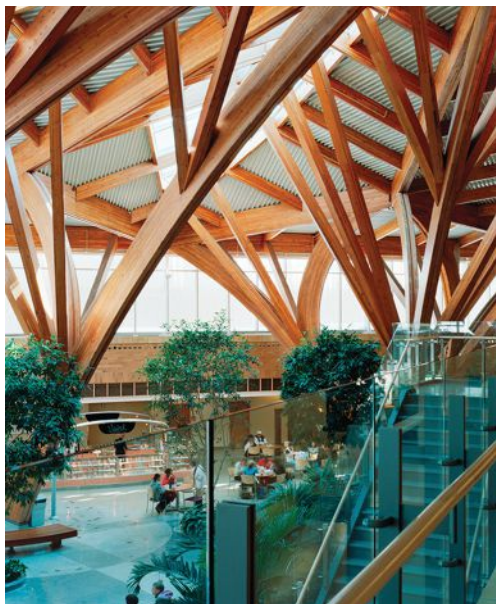
Credit Valley Hospital in Mississauga, Ontario, is one of an increasing number of healthcare facilities making use of exposed wood to create a warm, natural aesthetic that supports their healing objectives. Photo by Peter Sellar, Tye Farrow of Farrow Partnership, courtesy of naturallywood.com
