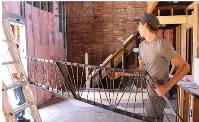
Students with the CUDC's design/REbuild project help renovate a vacant house
