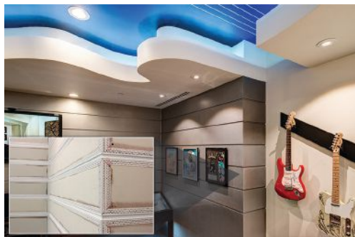
Reinforcing corners and reveal beads not only provide protection to drywall finishes but can also add aesthetic design elements.
