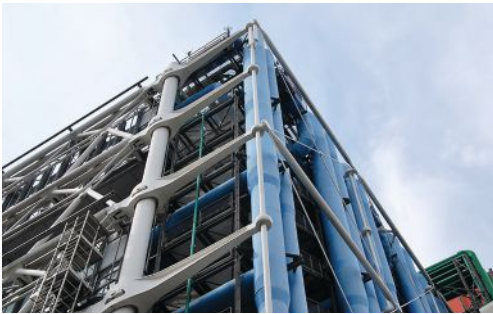
The Pompidou Centre in Paris, France was one of the first buildings in Europe to use architecturally exposed structural steel incorporating cast steel components. Photos courtesy of Terri Meyer Boake
