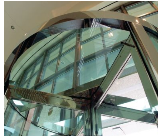
A four-wing, round drum, easy flow manual revolving door system is an excellent choice for energy efficiency and architectural appeal. Mechanical speed control and book-fold hardware for emergency egress are standard. Photo courtesy of Horton Automatics
