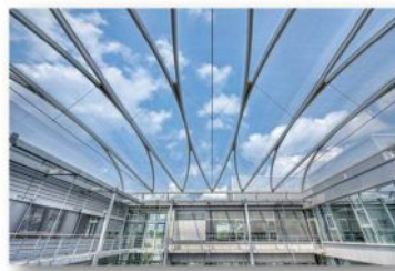
ETFE structures offer flexibility with design (Project: DWI Aachen by Carplus+Partner)
