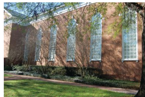
Acetylated Wood Carbon Negative Windows, Oakleigh USA. Photo courtesy of Accsys Technologies.
