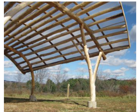
A 26-foot-tall, load-bearing black willow tree replaces a steel column at the Myrick Hixon EcoPark (top) in La Crosse, Wis., while branched timber frames a bandshell at Organic Valley's LaFarge, Wis., headquarters (above).
