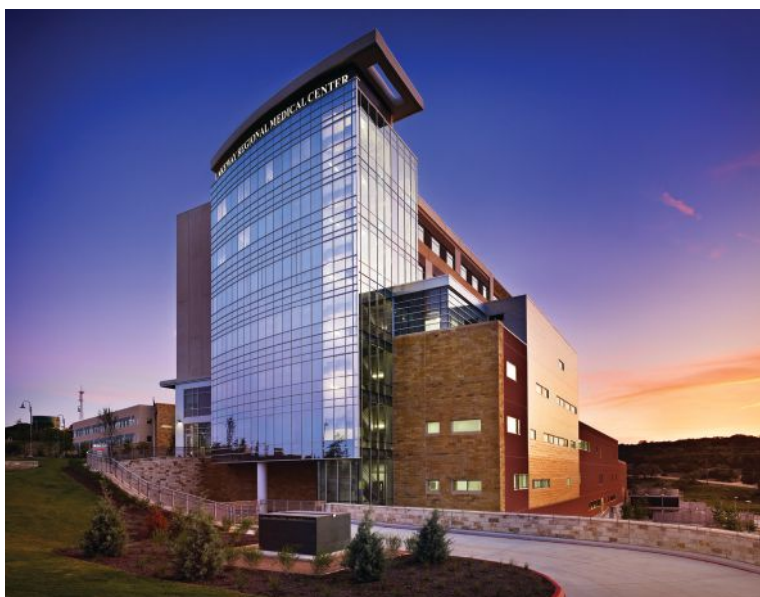
Designers maximized the tight, steep site by creating a tall and relatively narrow building, with dramatic natural views of the surrounding hill country. Photo Courtesy of Casey Dunn.
