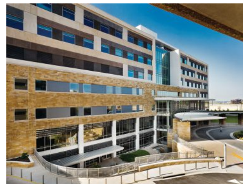
The exterior of the building is a combination of limestone veneer and precast concrete panels, which visually anchor the building to the site. Photo Courtesy of Casey Dunn.
