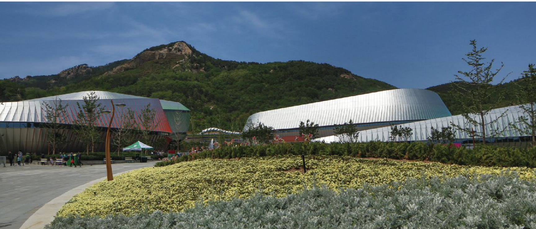
Opposite: A path leading past a yellow-accented section of one of the structures, with exterior planting displays on either side. Above: The building skins are assemblies of standardized metal components cut and bent into cylindrical, conical, and flat panels.
