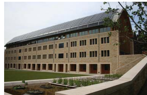
Education. Example: Kroon Hall, Yale School of Forestry & Environmental Studies, New Haven, CN., 60,000 sq. ft.
