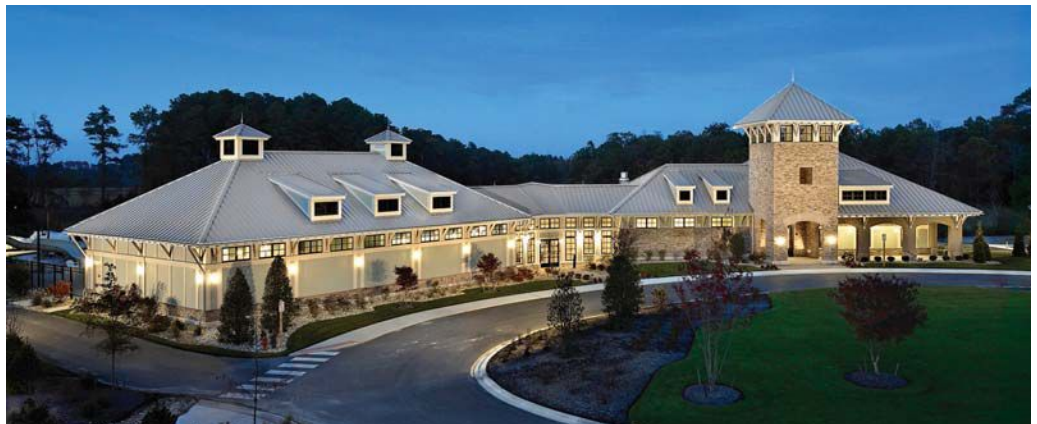
The Clubhouse at Bay Forest at Bethany Beach in Ocean View, Delaware, sports a metal cool roof, which reflects rather than absorbs the heat of the sun and reduces cooling costs for the building. Photo Credit: Petersen Aluminum
