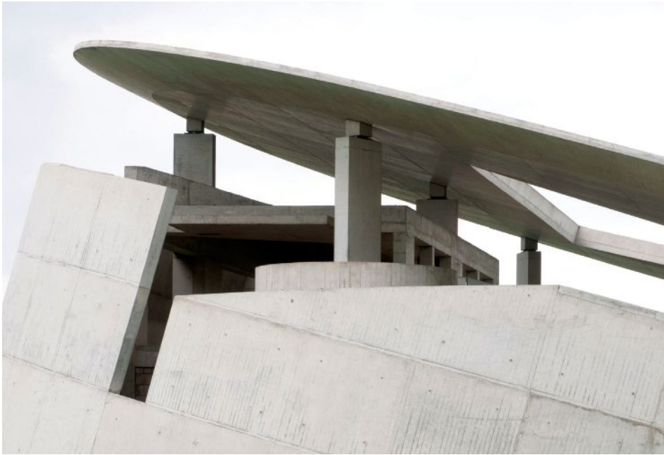
A detail showing a connection between the concrete base of the Musikerhaus and the concrete "crown" that graces the top of the building.
