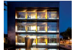
LOTT Clean Water Alliance in Olympia, Wash., by the Miller|Hull Partnership
