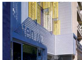
Step Up on 5th , a mixed-use project in Santa Monica, Calif., by Brooks + Scarpa Architects
