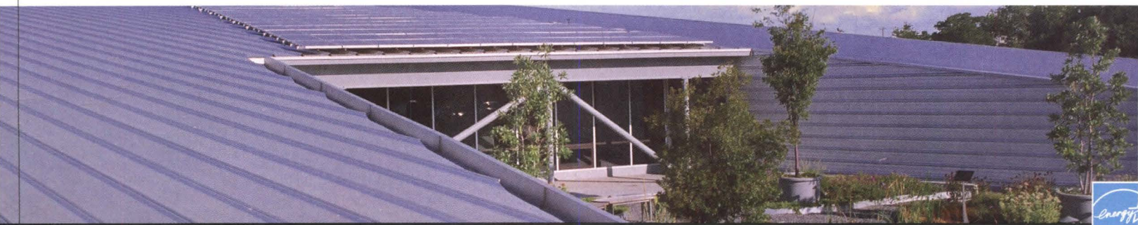
Bridges Center, Memphis, TN
