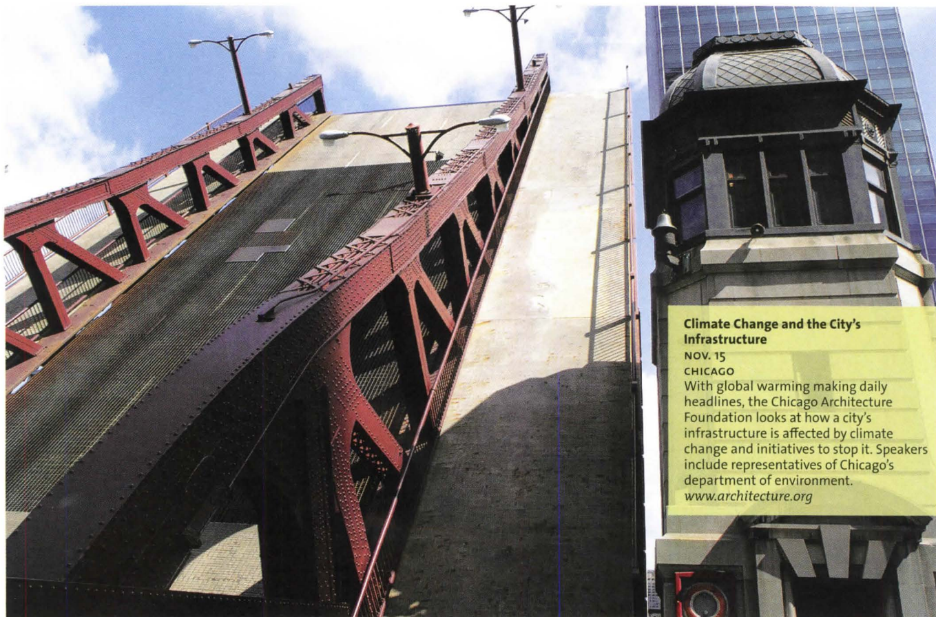
ANNE EVANS/COURTESY CHICAGO ARCHITECTURE FOUNDATION
