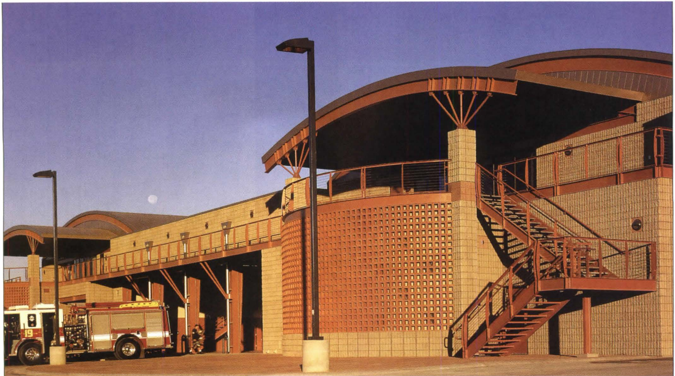
Air Rescue and Fire Fighting Station at Phoenix Sky Harbor Int'l Airport. Photo: Courtesy of National Concrete Masonry Association (For complete photo description, see online material).
