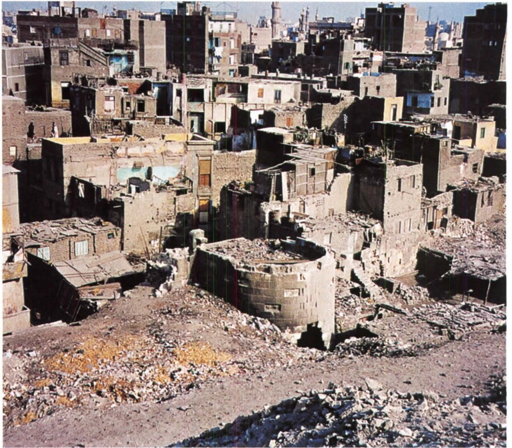
THE NEARLY MILE-LONG, TWELFTH-CENTURY ABBUYID WALL FOLLOWING THE REMOVAL OF 35 CUBIC FEET OF RUBBLE (PREVIOUS PAGE) FORMS THE SOUTHERN EDGE OF CAIRO'S NEW AZHAR PARK; SEVERAL TOWER FORTIFICATIONS WERE UNEARTHED DURING THE EXTENSIVE TEN-YEAR RESTORATION PROCESS (ABOVE).
