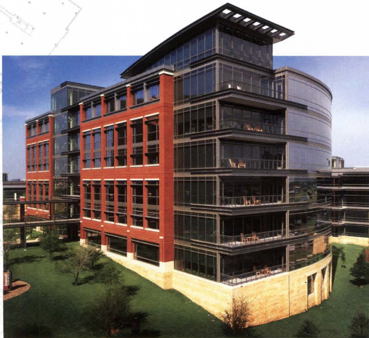
RadioShack World Headquarters Riverfront Campus VRE 1-46 (Viracon Radiant Low-E) Fort Worth, Texas Wes Thompson Photography
