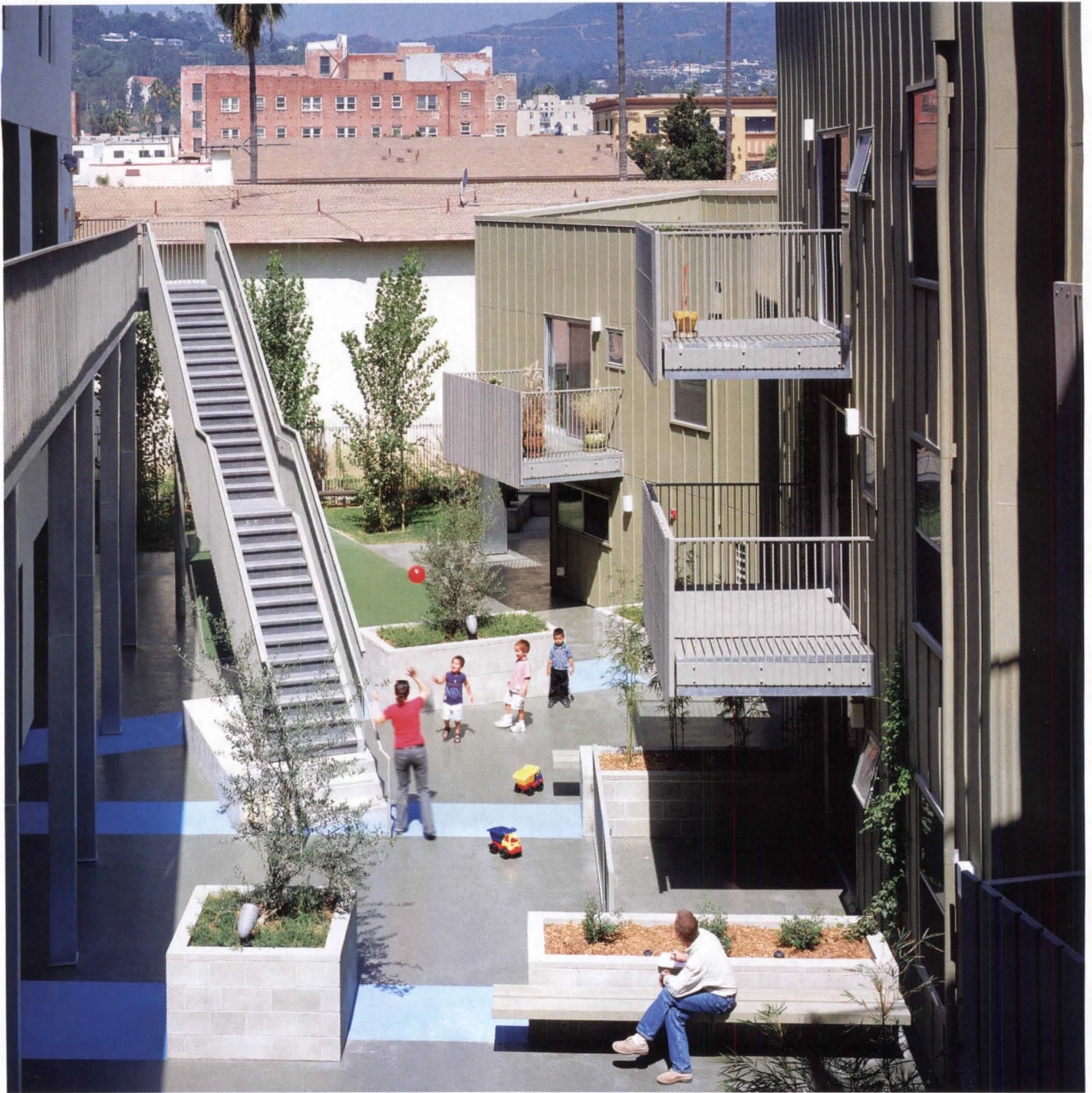
At Harold Way Apartments, a 50-unit complex in Hollywood, Koning Eizenberg negotiated between economic moves and the things that “make it nice to get up in the morning” and “hang around on the weekend”: a zigzagging courtyard and cement-board-and-wood-batten cladding.
