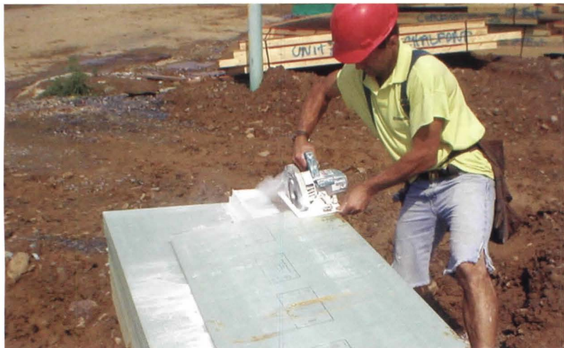
Gypsum board area separation wall liner panels can easily be trimmed with a power saw or knife to meet any size requirement.
