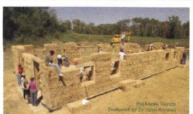
Building a Straw Bale House: The Red Feather Construction Handbook
