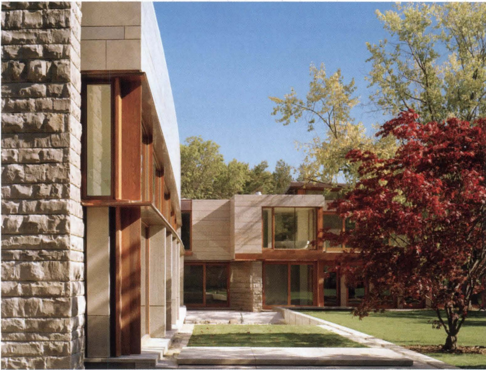
SHADE TREES AND A REFLECTING POOL DEFINE THE HOUSE'S REAR COURTYARD (ABOVE), WHICH NESTLES OUTSIDE THE FAMILY ROOM AT THE JUNCTION POINT OF THE "L." LIMESTONE IN SMOOTH AND RUSTICATED FINISHES LENDS TEXTURAL VARIETY.
