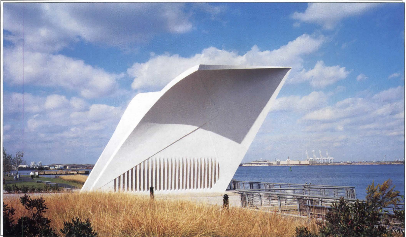
granite profiles cut to resemble the borough’s honored victims are artfully backlit at night by in-ground uplights located on the other side of the wall. Serving as marker lights, small one-inch-diameter LEDs trace the base of the memorial’s interior (top, left).
