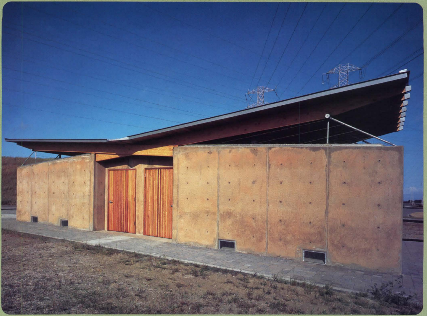
Rendered in cast-in-place concrete walls and custom cedar-batten doors, the restrooms are protected by a butterfly roof with a standing-seam metal deck on cedar rafters and galvanized-steel pipe framing
