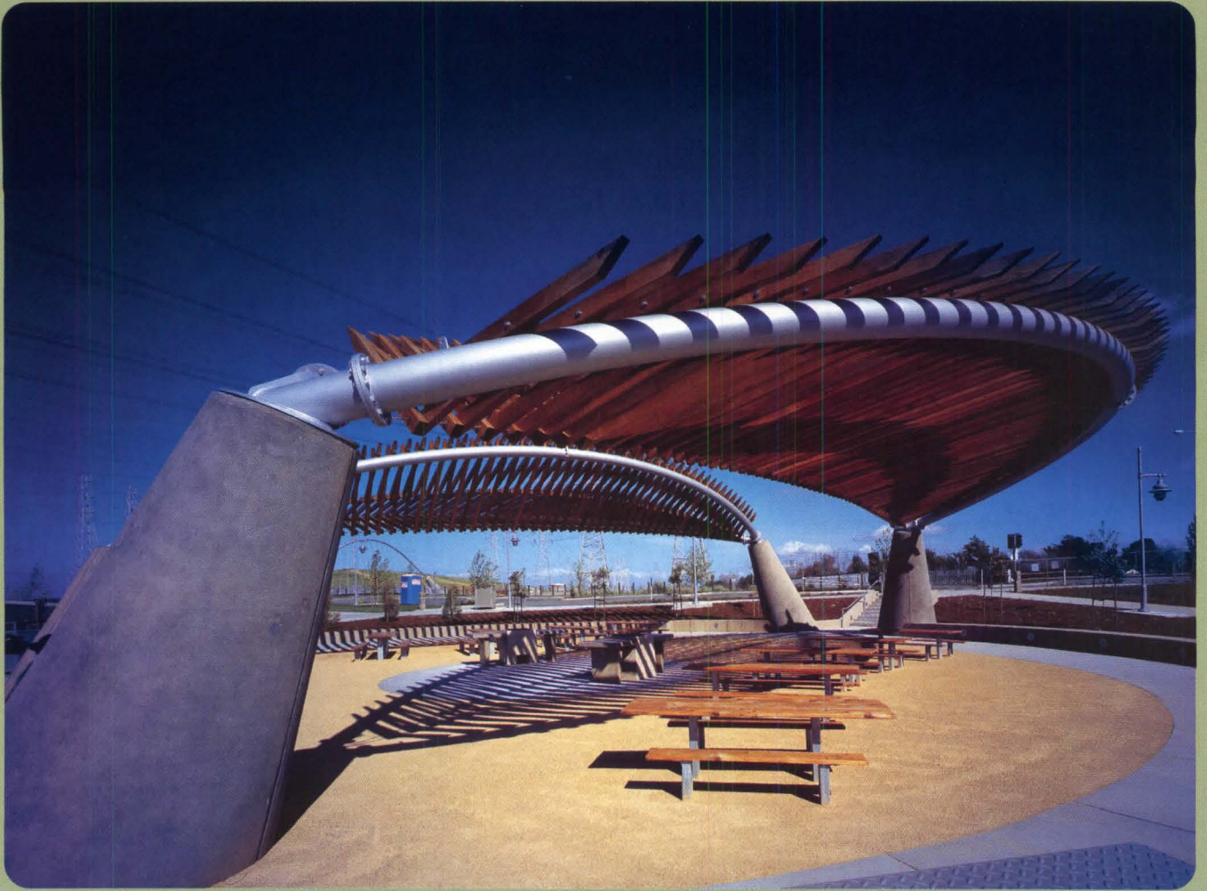
For picnickers, western red cedar slats resting on bowed steel members provide a shade canopy, jutting out to 18 feet at their widest point. The pedestrian bridge is visible beyond the picnic area.
