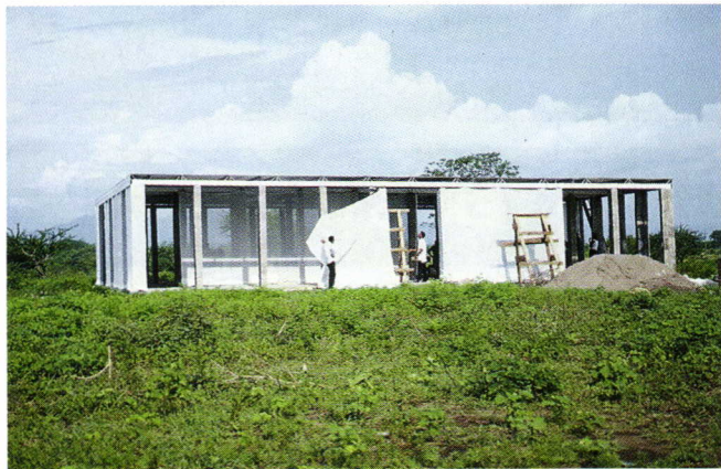
Built by local residents, Jae Cha's community center-church (left) in Marcovia, Honduras, is framed in steel-reinforced concrete blocks and sheltered by a corrugated metal roof; a mesh fabric commonly used for agricultural shading forms interior and exterior walls as needed. M. Scott Ball's Moseley House (right) in Atlanta is the result of a design-build initiative that engages student interns and homeowners.
