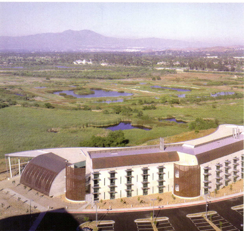
The lab-and-office building's layered envelope provides degrees of privacy and transparency to occupants, as well as control of heat and light transmission. Copper and stainless-steel sunscreens animate the southwestern exposure (top), while the view to the east is of wetlands and the San Gabriel Mountains (above).
