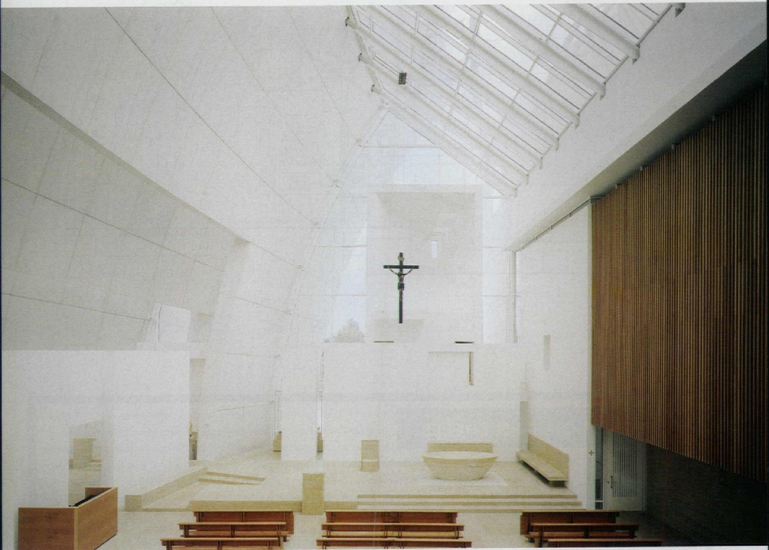
The nave is clad in travertine from nearby Tivoli. Along one side of the space, a slatted hemlock panel conceals a second-story walkway.
