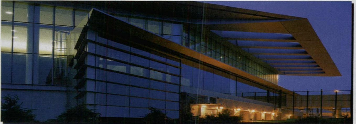
Aerodynamic eaves project from glass-finned curtain walls at the converging masses of the main terminal and the long concourse pier (top). The powerful corner was to contain an elegant lounge; airport authorities later decided to partition it off as a duty-free shop.
