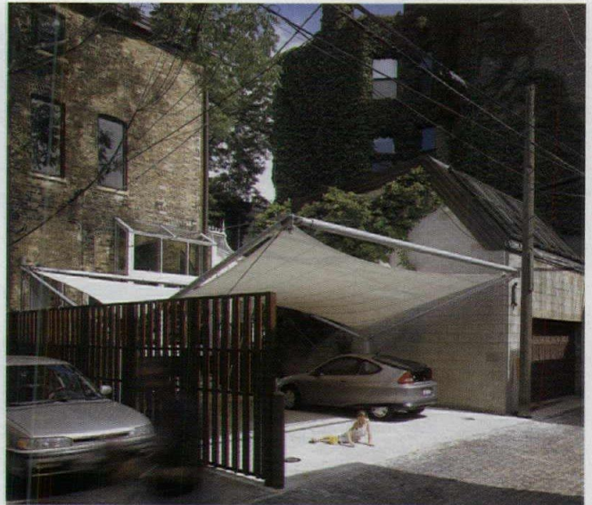
The white carport, whose brightness Studio Gang emphasized by whitewashing the adjacent wall, contrasts with the brick of the townhouses around it (above). The tight double curvature of the canopy can be seen clearly in section (below).
