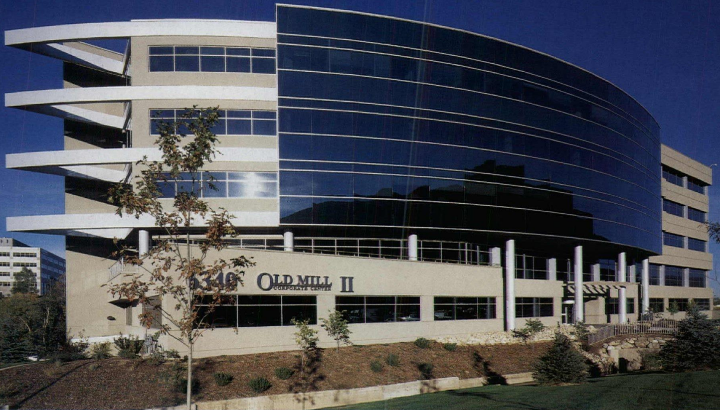
Old Mill II Corporate Center, Salt Lake City, UT, VCBO Architecture
