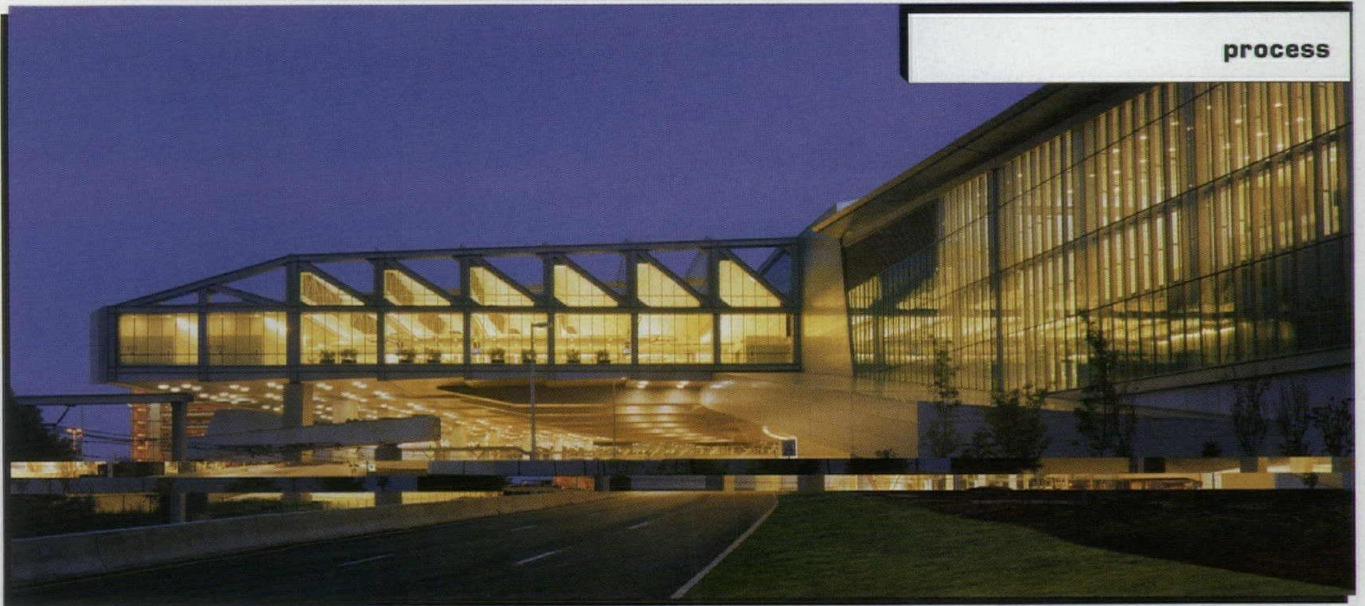
The passenger drop-off is spanned by 190 feet of brightly illuminated, silvery composite panels, supported by a large truss above it. The underside of the carport features eight soffited bulges showing where conveyor belts rise to the baggage-claim area. The narrow main terminal is highly transparent, admitting light and allowing ample views between programmatic elements and to the outside.
