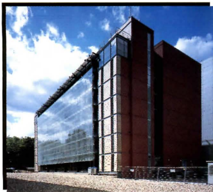
The Darwin Centre's south façade allows maximum daylight penetration, aiding the microscope work inside while venting against heat gain (above left). Half the building is cold storage for some 20 million biological specimens suspended in ethanol-filled jars (above right).
