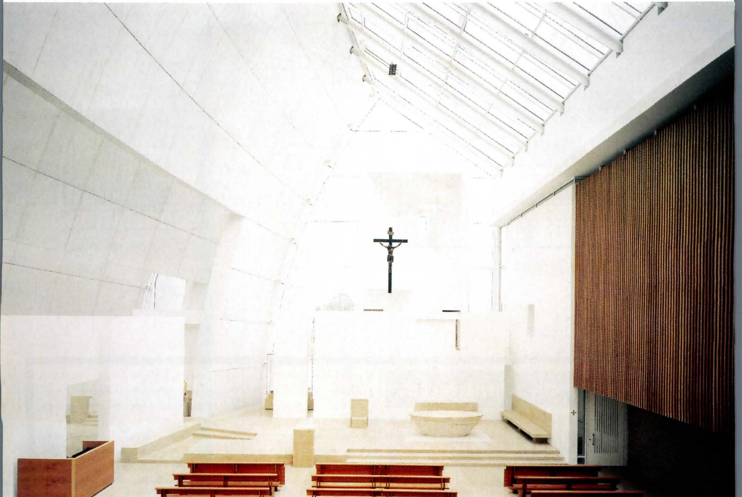
The nave is clad in travertine from nearby Tivoli. Along one side of the space, a slatted hemlock panel conceals a second-story walkway.
