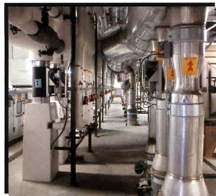
Anshen + Allen used a “wolf in sheep’s clothing” approach to the Contained Research Facility; it’s modeled on a simple barn (above left). Inside is the “hot rod,” the equipment that allows the building to operate as a biosafety-level-3 research greenhouse (above right).
