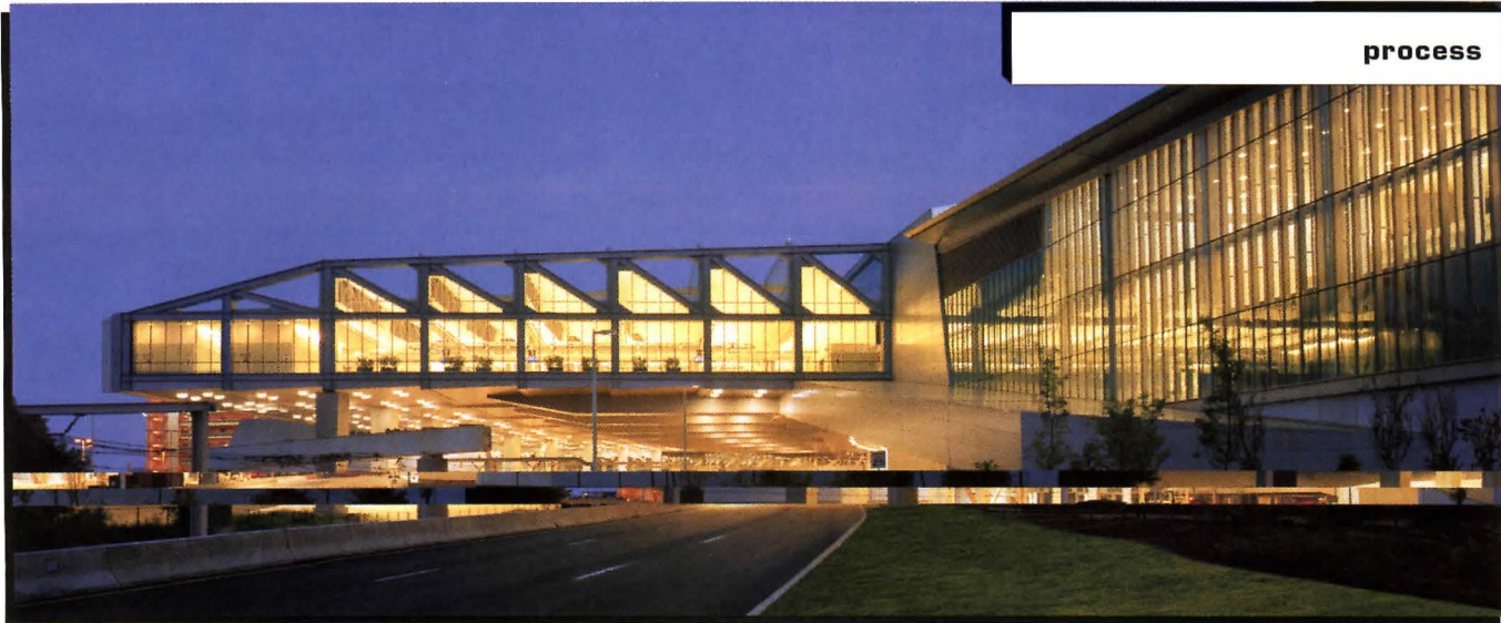
The passenger drop-off is spanned by 190 feet of brightly illuminated, silvery composite panels, supported by a large truss above it. The underside of the carport features eight soffited bulges showing where conveyor belts rise to the baggage-claim area. The narrow main terminal is highly transparent, admitting light and allowing ample views between programmatic elements and to the outside.
