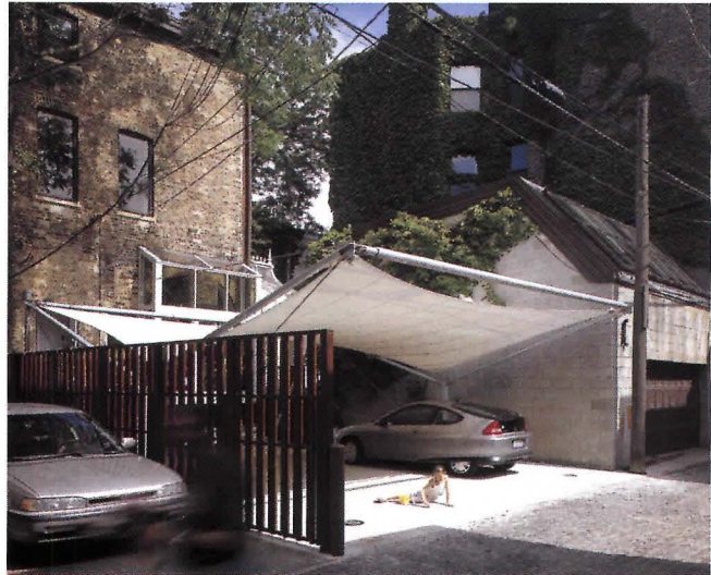
The white carport, whose brightness Studio Gang emphasized by whitewashing the adjacent wall, contrasts with the brick of the townhouses around it (above). The tight double curvature of the canopy can be seen clearly in section (below).
