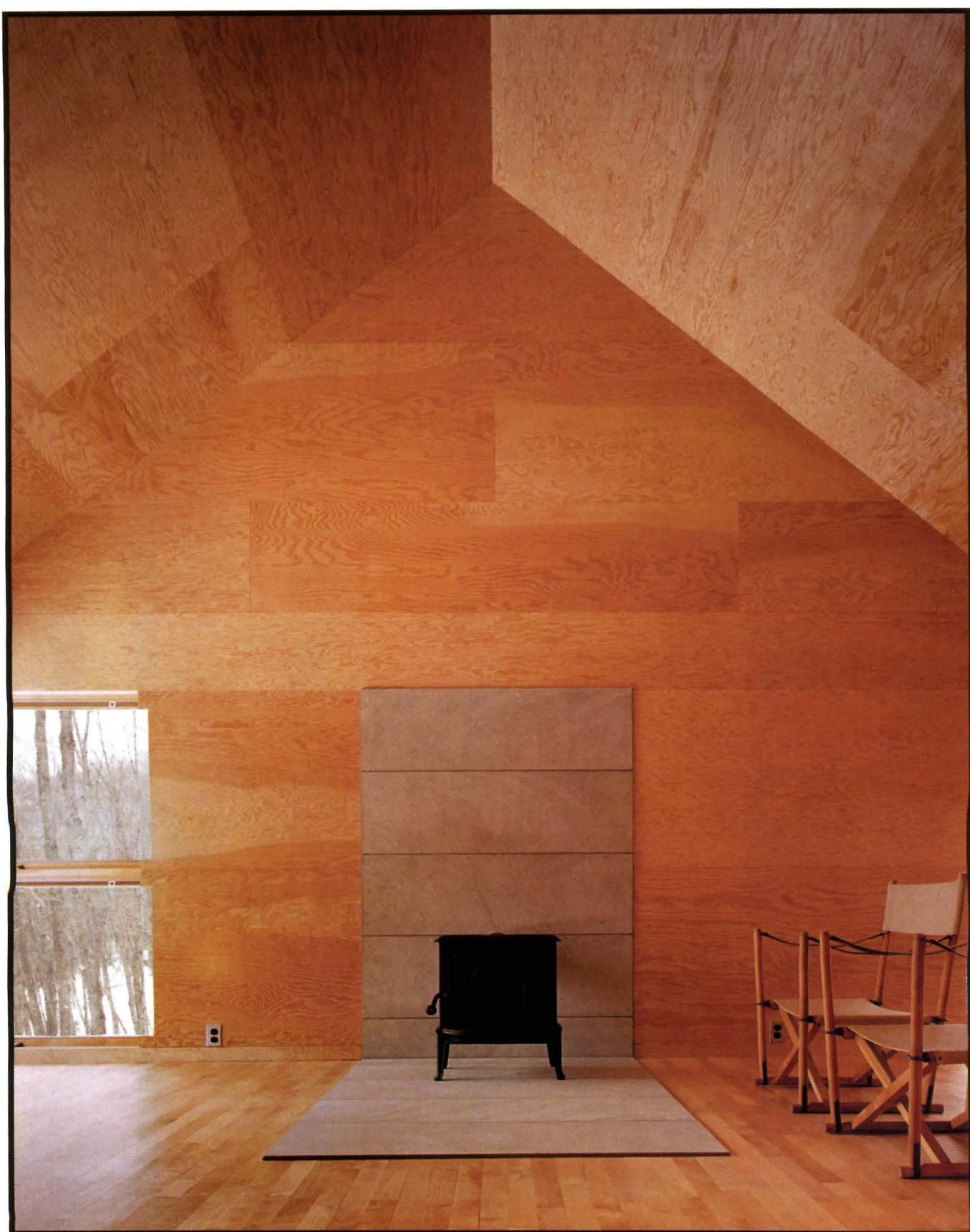
Maison Goulet sits in an undisturbed stand of birch and maple trees about an hour drive north of Montreal (facing page). Lightly stained half-inch-thick plywood lends both log-cabin warmth and a rigorous order to the interior spaces (above). The dramatic but spare office area centers on a wood stove and limestone slabs.
