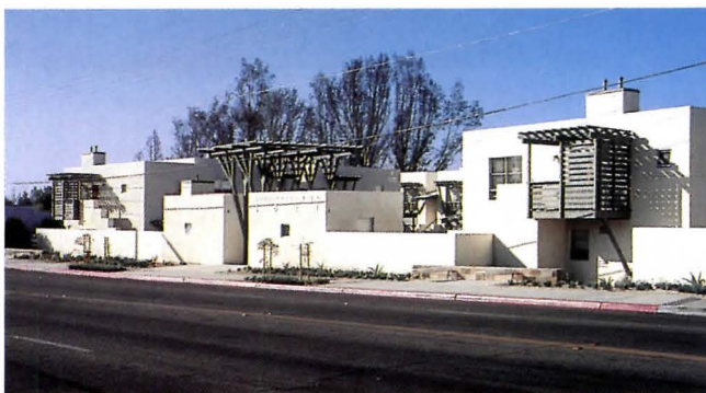
At Eucalyptus View, semiprivate porches and patios encourage residents to occupy the zone straddling individual units and a communal courtyard (top). An oversized pergola emphasizes the pedestrian entry (above).
