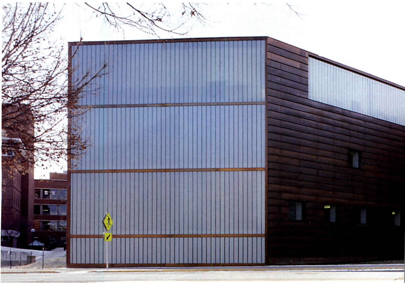
The channel-glass ends of the school's wings are signature features, even more so after sundown.
