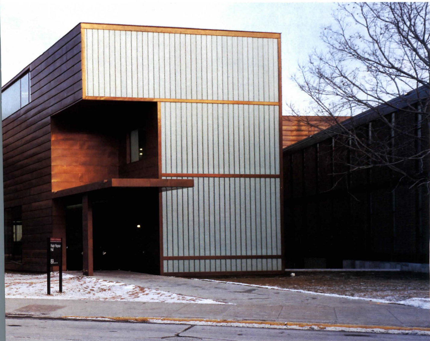
Clad in copper sheet and channel glass, Holl's structure joins the existing school (at right) to form the Ralph Rapson College of Architecture and Landscape Architecture, named for the revered former dean. The canopy marks the new main entrance.
