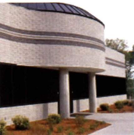
oca-Cola Bottling Company of Northern New England, Inc., Londerry, NH chitect of Record/Engineer: Stahlman Engineering Corporation, New London, NH cent Panels: 3 5/8" x 23 5/8" x 3 5/8", #M115, #M1428 ish: Tudor
