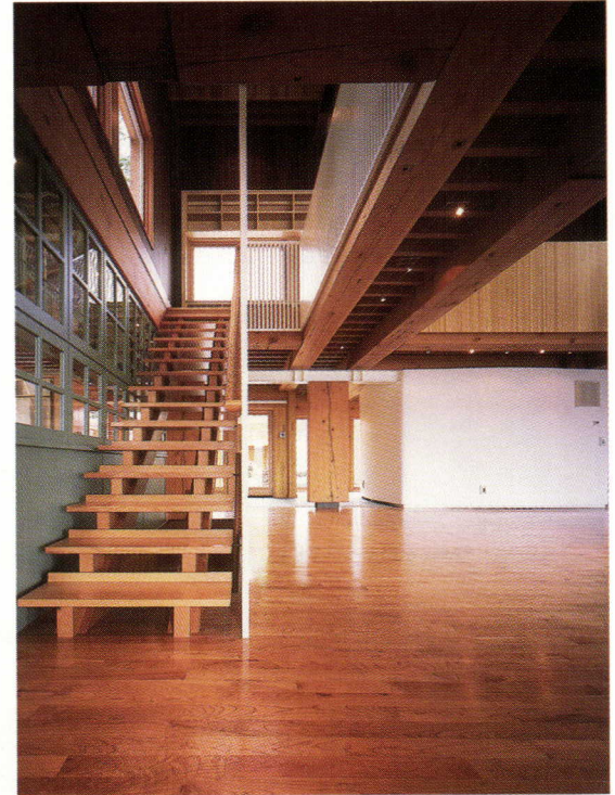
The stair screen (above) is only an inch and a half thick and stands 13 feet tall. The screen and stairs are separated by a small space to ensure they are two distinct elements.
