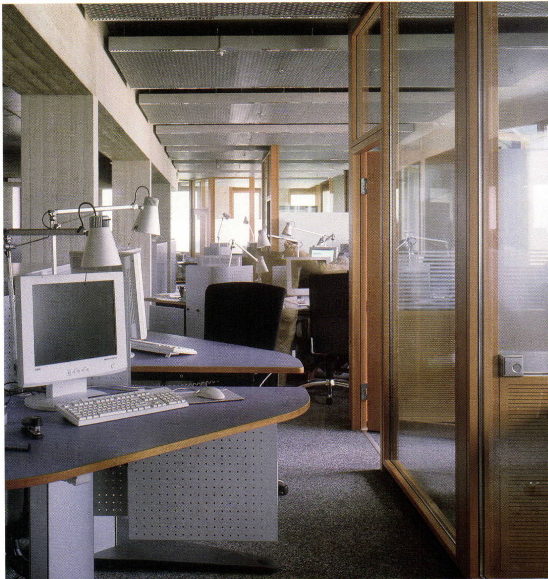
The office interiors feature "cockpit" partitions of Oregon pine and etched acoustical glass with thin steel profiles and a three-layer acoustic panel. A stainless-steel box contains a thermostat to measure ambient temperatures (opposite, center). Custom-made ceiling elements integrate lighting, cooling coils, and acoustical insulation inside a slotted steel frame (opposite, top right).
