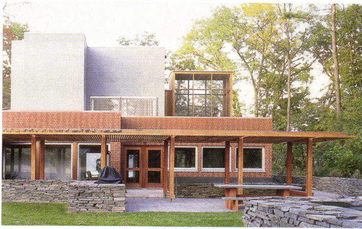
The library volume is differentiated from the main house with slate cladding (above) and a shift in section that creates an overhang to the north (section, top). A detail drawing of the library's slate façade (right) shows the careful construction of the façade and the connection to the roof below.
