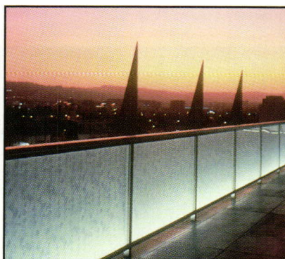
Petersen Museum Exterior Railing
