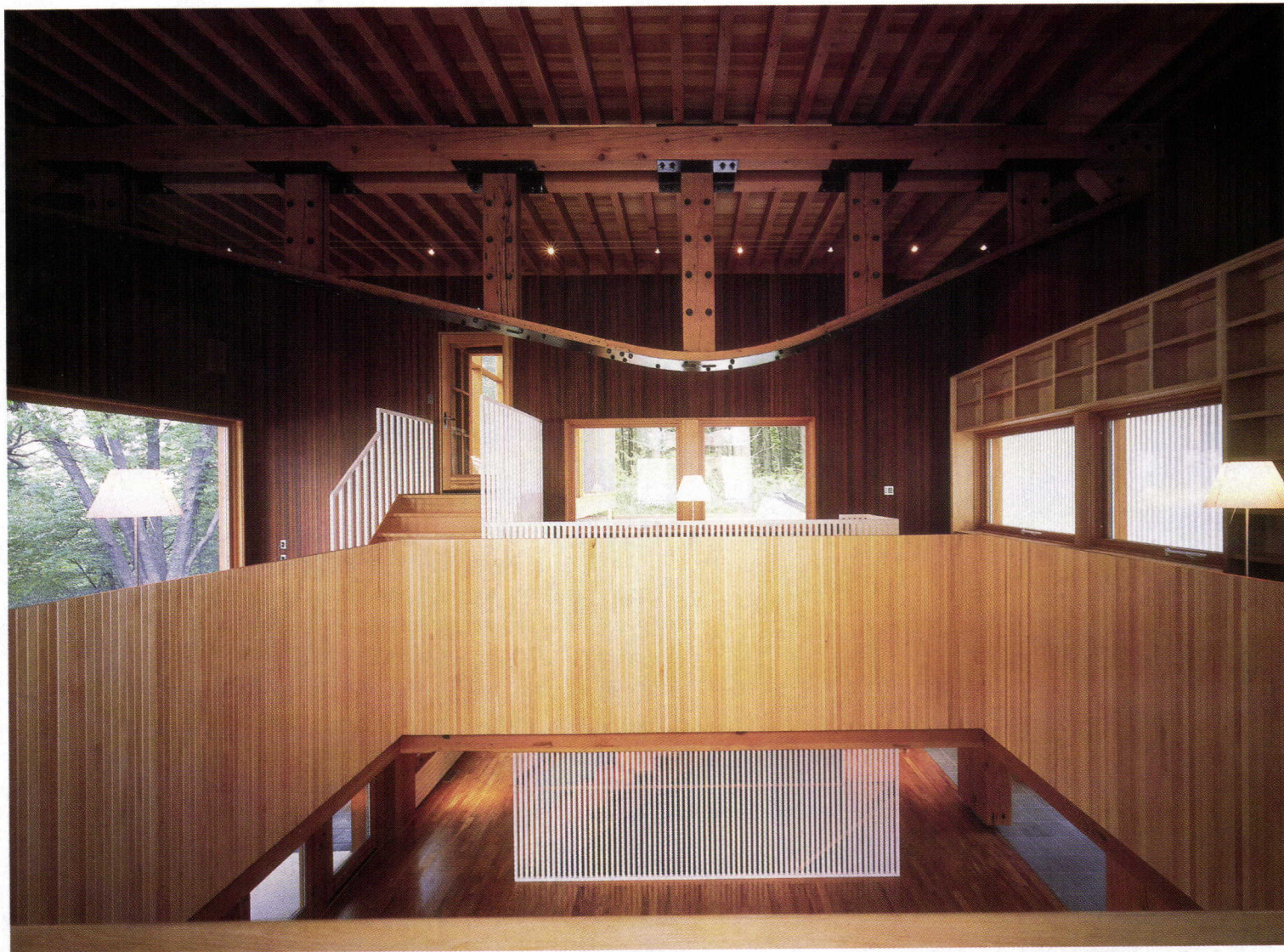
The library (above) boasts a number of species of wood, including recycled redwood siding, basswood slatting around the interior opening, and new and recycled Douglas fir in the roof structure. The design uses eight distinct species in all.
