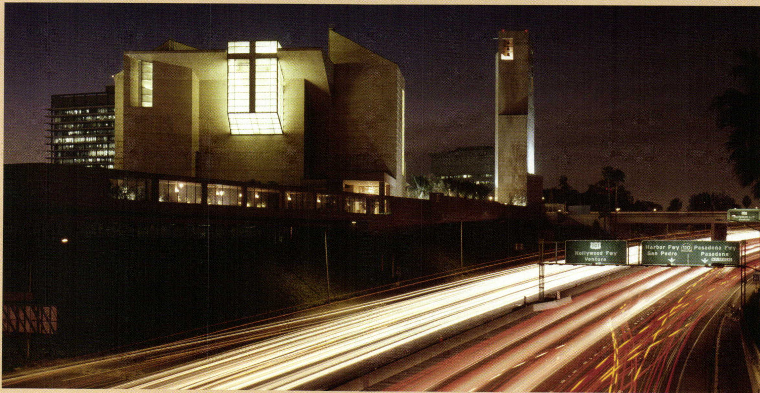
A focal point for L.A.'s maturing cultural corridor, José Rafael Moneo's recently completed Cathedral of Our Lady of the Angels sits on a 5.6-acre site overlooking the Hollywood Freeway. Moneo likened the infamous road to a river that connects Los Angelenos to each other.
