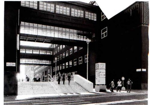
Near a corner of the university square, skyways preserved from former Pirelli factory buildings on the site connect the units of the humanities department.
