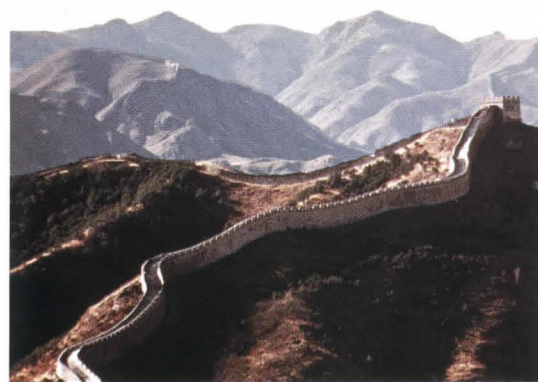
R. M. Schindler's Kings Road House and Studio (top), completed in 1922, suffers from water damage, a leaking roof, and failure of some structural elements; increased tourism and development surrounding the Great Wall of China (above) threaten its fragile landscape.
