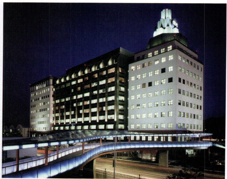
Façade from Riverside Drive
