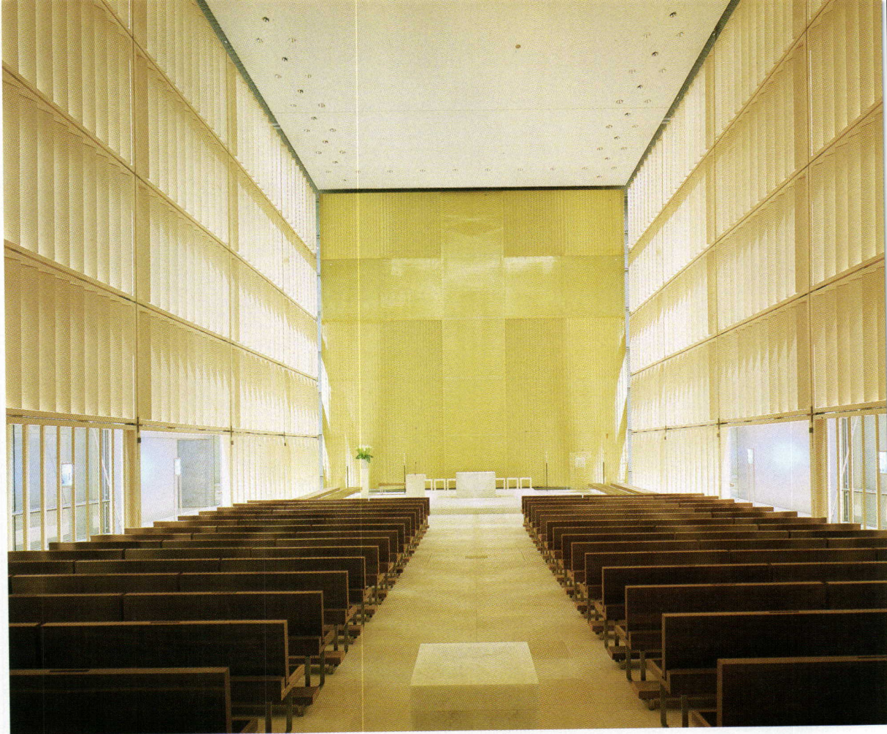
Behind the altar, four different weaves in the fine golden metal mesh create a subtle image of the cross (above, at center). The upper four layers of angled maple louvers along the nave direct sunlight toward the altar, while the lowest layer faces the opposite direction, allowing churchgoers
