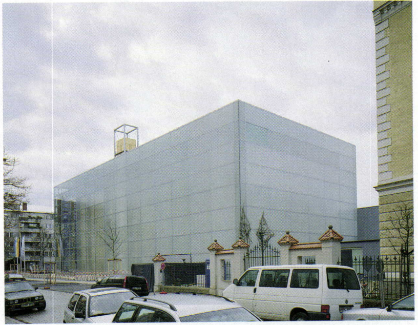
Except on holy days, the massive blue portals of Munich's Church of the Sacred Heart (preceding pages) are left closed; otherwise, parishioners enter via the two small inset doors (facing page). Clear silhouettes of nails etched into the blue glass are arranged in letters that spell out the story of Christ's Passion according to the Gospel of St. John. The glass panels that clad the building are transparent when close to the portals, but grow increasingly cloudy as they near the altar at the rear of the church (above).
