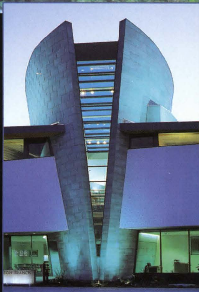
Project: Robertson Branch Library City of Los Angeles Architect: Steven Ehrlich Architects
