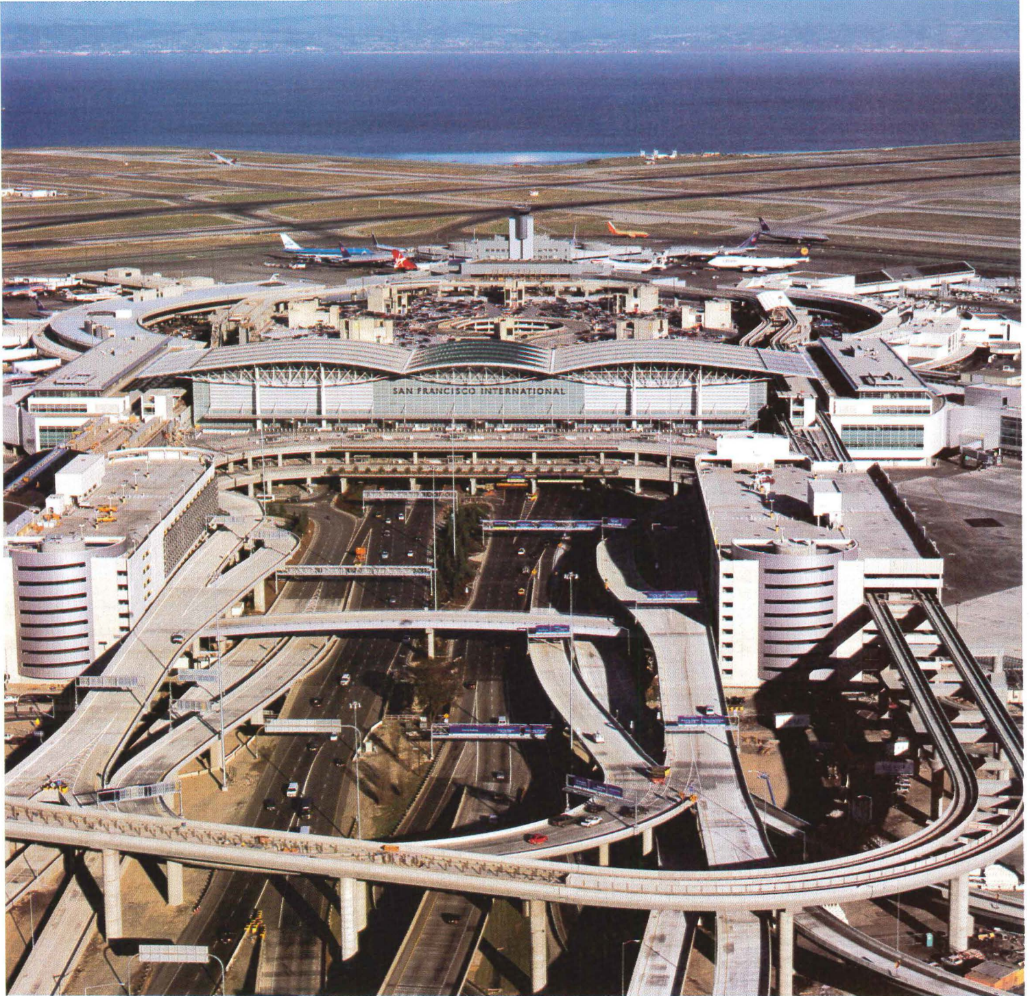
Site The tangled web of overpasses, light rail and BART tracks, and two parking garages in the foreground are the work of separate firms working under only the loosest design supervision. The airport has now filled every meter of available land, and the International Terminal closes the diagrammatic circle of existing terminals to complete the master plan.
