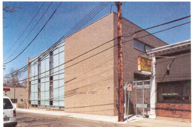
Berke employs a curtain wall on the façade facing quiet Crown Street (above), where diners and bungalows are more prevalent than museums and university buildings. A new ramp and stair (top) give access to the rear of the former community center. The stair is visible at the end of an alley (facing page) that leads from the small midblock courtyard to Crown Street.
