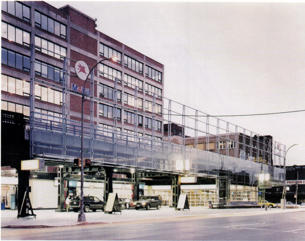
The Chelsea Carwash's 202-foot façade (above) is a simple tube-steel-and-glass armature attached to the abandoned New York Central Line freight tracks. The glass behaves like a billboard: The Carwash advertises its services by making them clearly visible from the street, and attracts attention with the reflection of the Hudson's afternoon light. The glass sheets are affixed to the steel structure (facing page) with patch plates. Front and rear plates (with neoprene disks) clamp the glass into place and are bolted to the tube steel.
