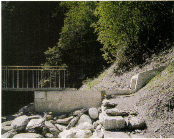
The Suransuns footbridge hovers above the rocky banks of the Hinterrhein (top left and right, and facing page), linking the ancient Via Mala hiking path to a larger network of trails. The steel ribbons which give the bridge its strength run beneath the granite pavers and terminate in tensioners anchored into landside concrete abutments (bottom left and right).
