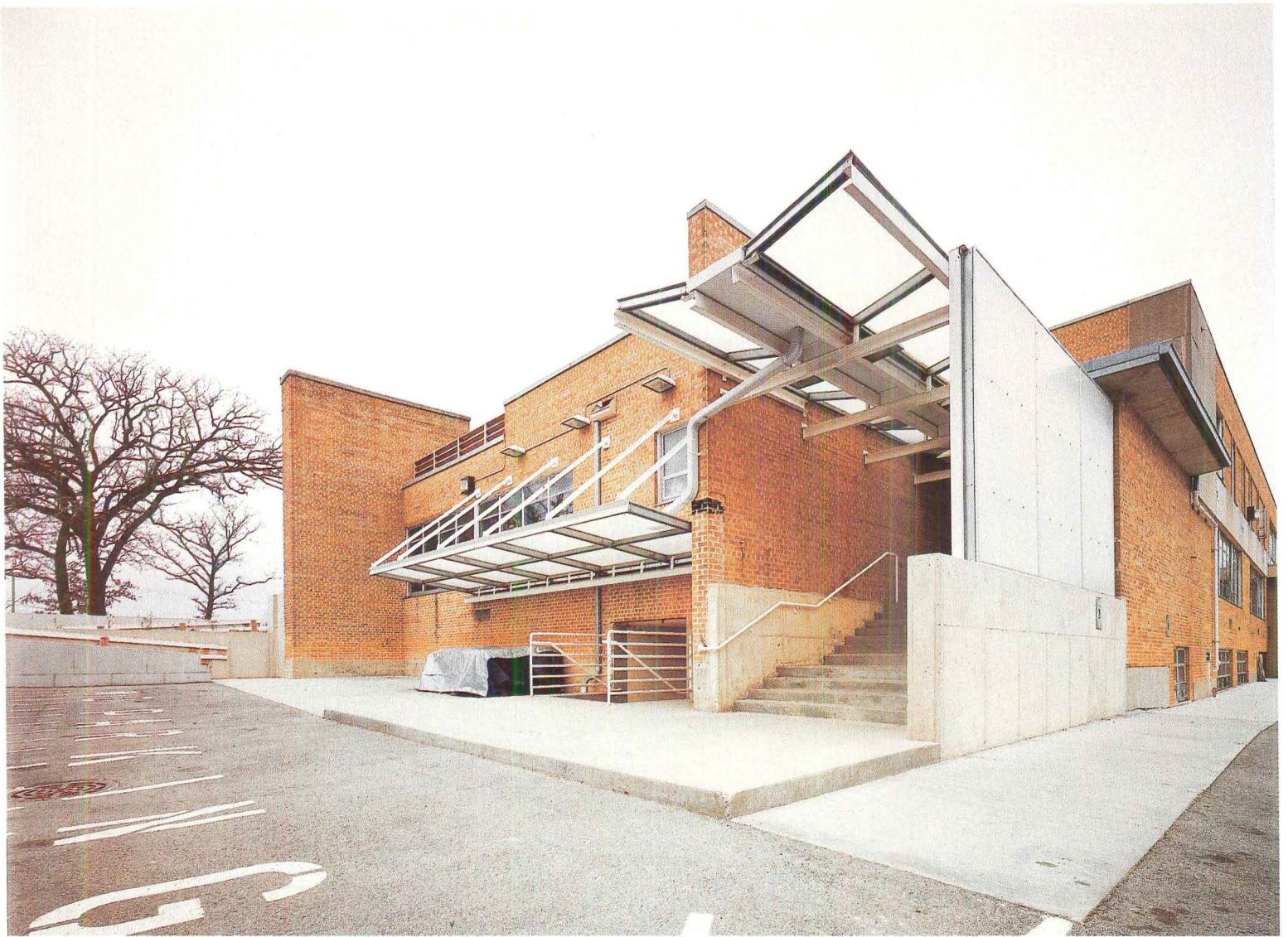
The only addition to the exterior is a canopy (above) made of galvanized steel and a translucent plastic commonly used in greenhouses. Students enter under the canopy (below left) up a flight of stairs, where the hallways are lined with cubbies and benches (below right). Butterfly-shaped false skylights, lit from behind, simulate daylighting in the lunchroom (facing page, top), the art room (middle), and the library (bottom). A large pivoting door allows the art room to expand into the adjacent area. This device fulfills the Montessori principle that says adjustable spaces are preferable to static ones.
