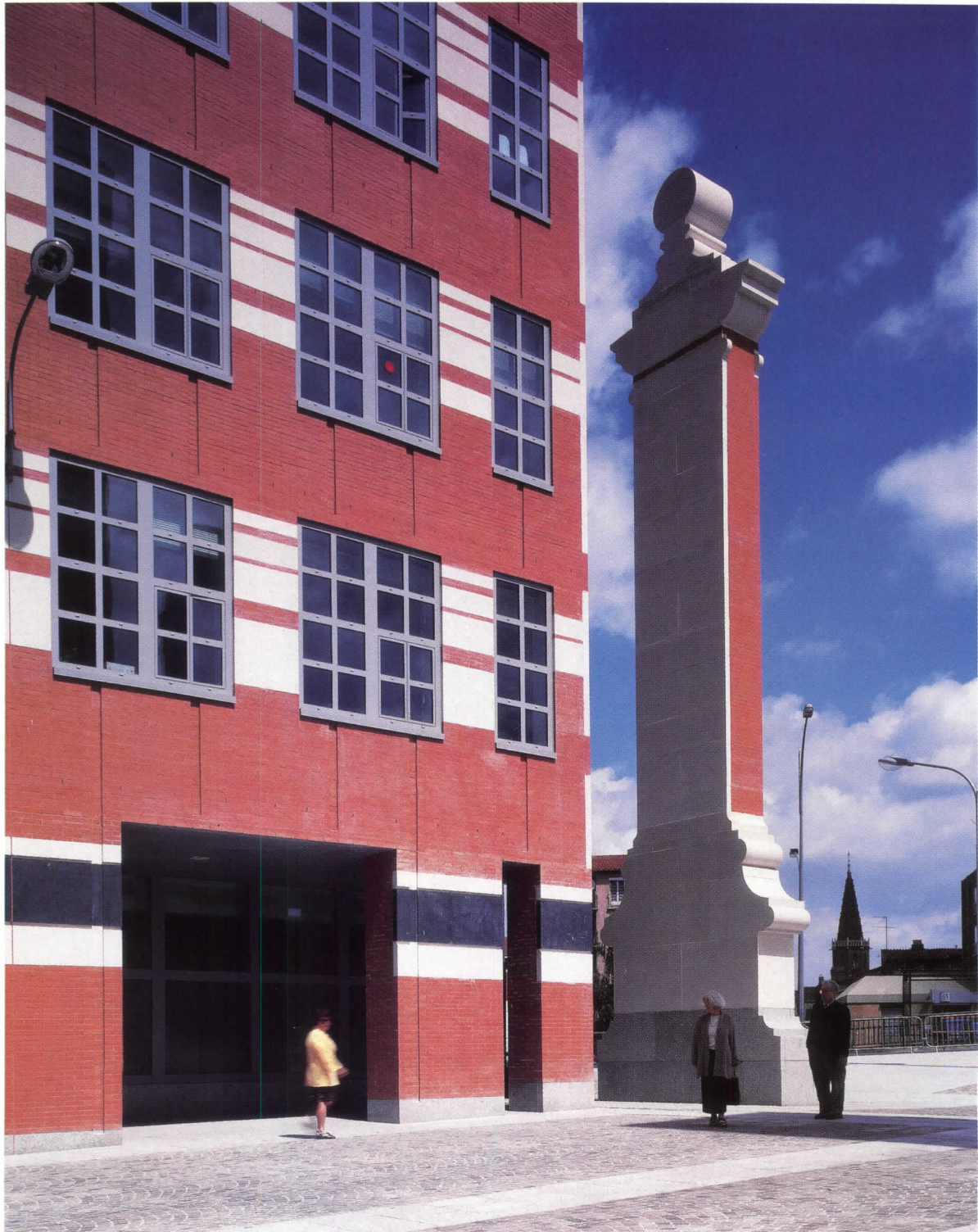
Arcades (above) line the public passage between the two wings. Above, the windows' fat mullions evoke the fenestration of a Renaissance mansion in Toulouse ( fig 7 ). The blank limestone surface at the rear of the column (at right) exemplifies how VSBA flattens iconography and ornament.
