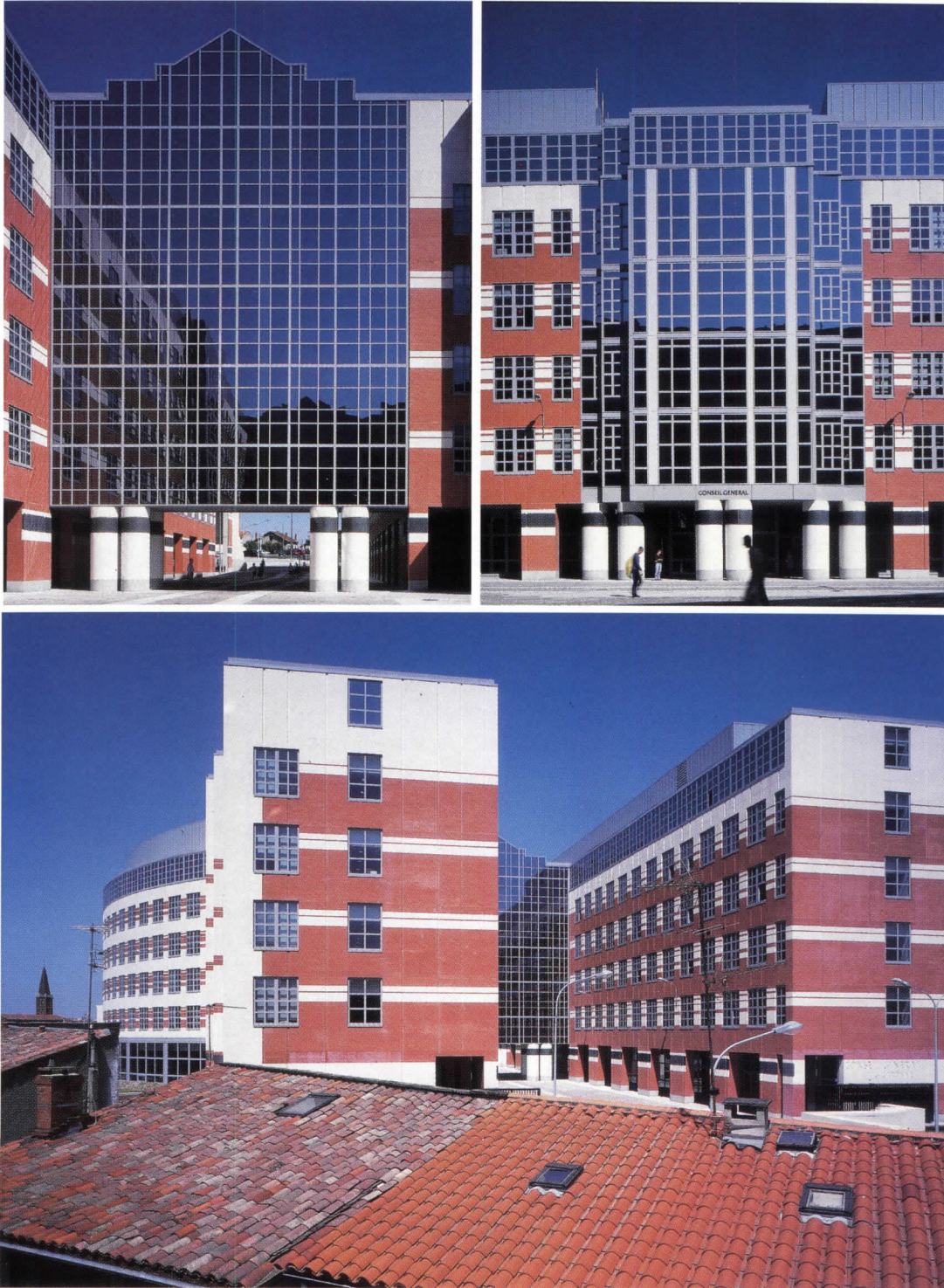
The pointedly simple south facade (above) backs up to traditional red-tile-roofed row houses. As on the north side of the building, the streetlike space between the wings echoes the form and original purpose of the Uffizi in Florence. Instead of framing a view of the Arno River, however, the two identical glazed bridges (above and top left) between the wings bound a central courtyard. Another expanse of glass (top right) marks the entrance to the assembly hall in the central courtyard. At the base, VSBA parodies its own signature center column by doubling it.
